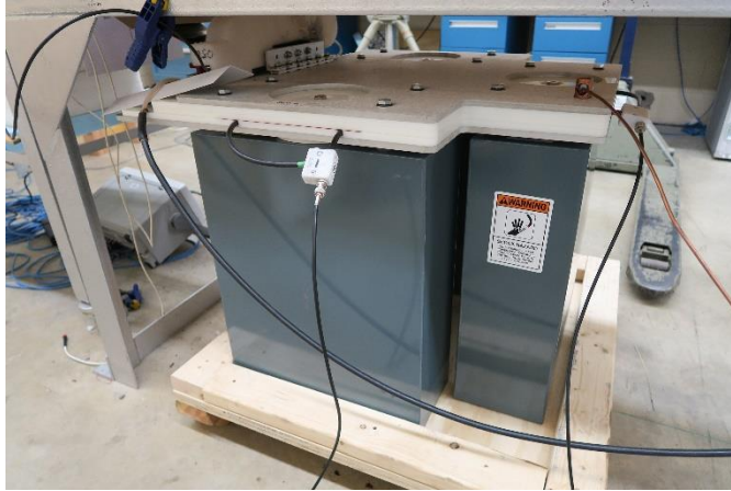
Fig. 5 New ICAR Bioenergy capacitor bank
