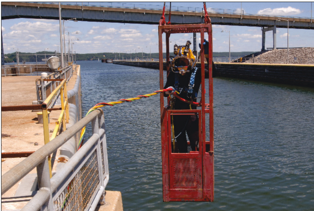
Figure 5. USACE diver inspection of Pickwick Lock, near Counce, TN.
