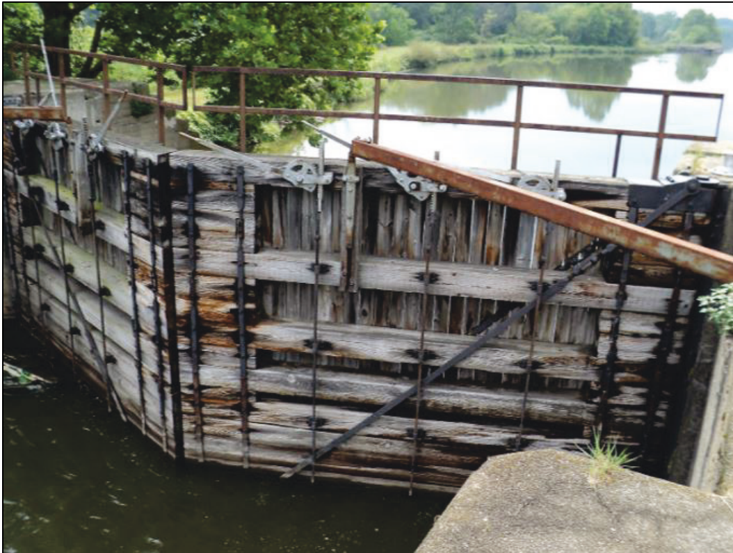
Figure 3. Wooden miter gate, Lock 16, Hennepin Canal, near Geneseo, IL.
