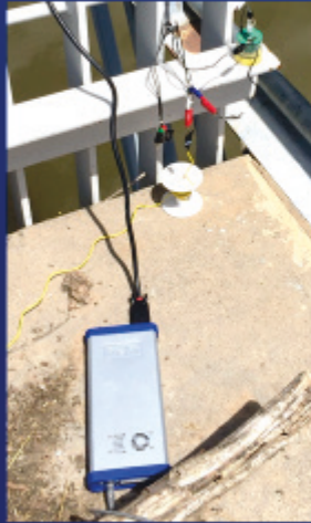
EIS test using portable potentiostat from Ivium
