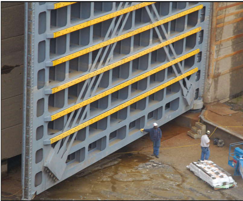
Figure 6. Downstream miter gate leaf installed at Markland Locks and Dam, Ohio River.
