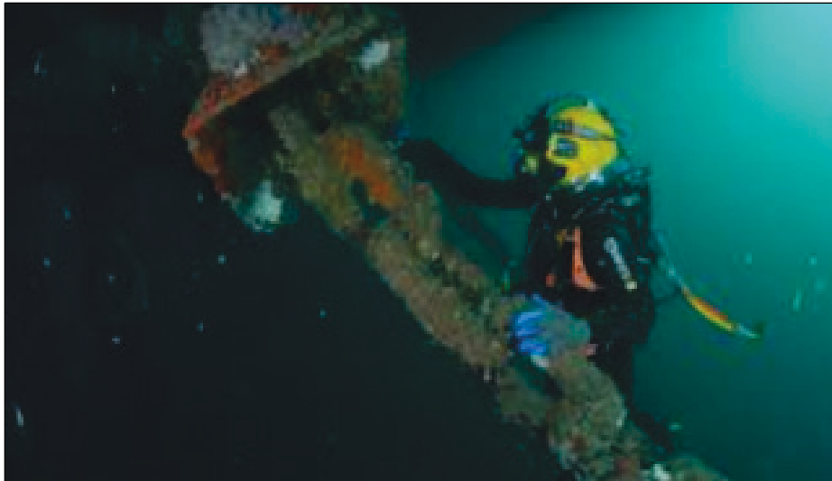
Figure 8. Diver visual inspection for corrosion.
