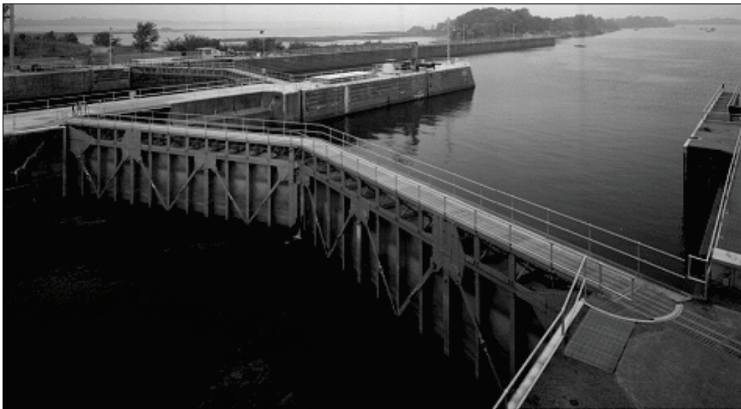
Figure 2. Typical hydraulic steel structure miter gate, opening upstream.
