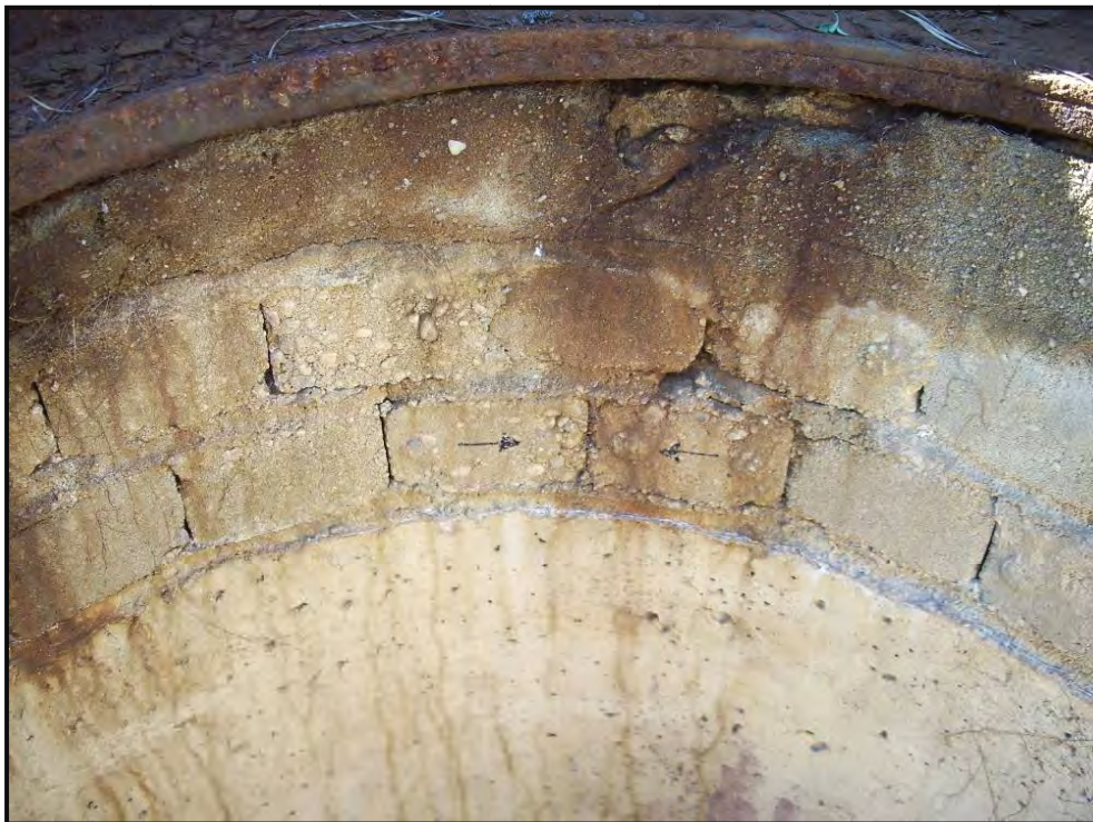
Figure E-10. Bulkhead to Shelter 216 Power Bunker (Arrows Indicate Location of \alpha -Radiation Contamination on Grout).
