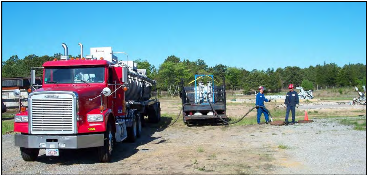
Figure E-4. Pumping and Filtering Water from Shelter 208 Power Bunker.
