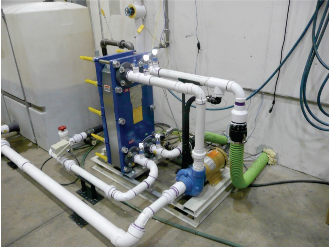
Figure 13. Isolation heat exchanger skid.
