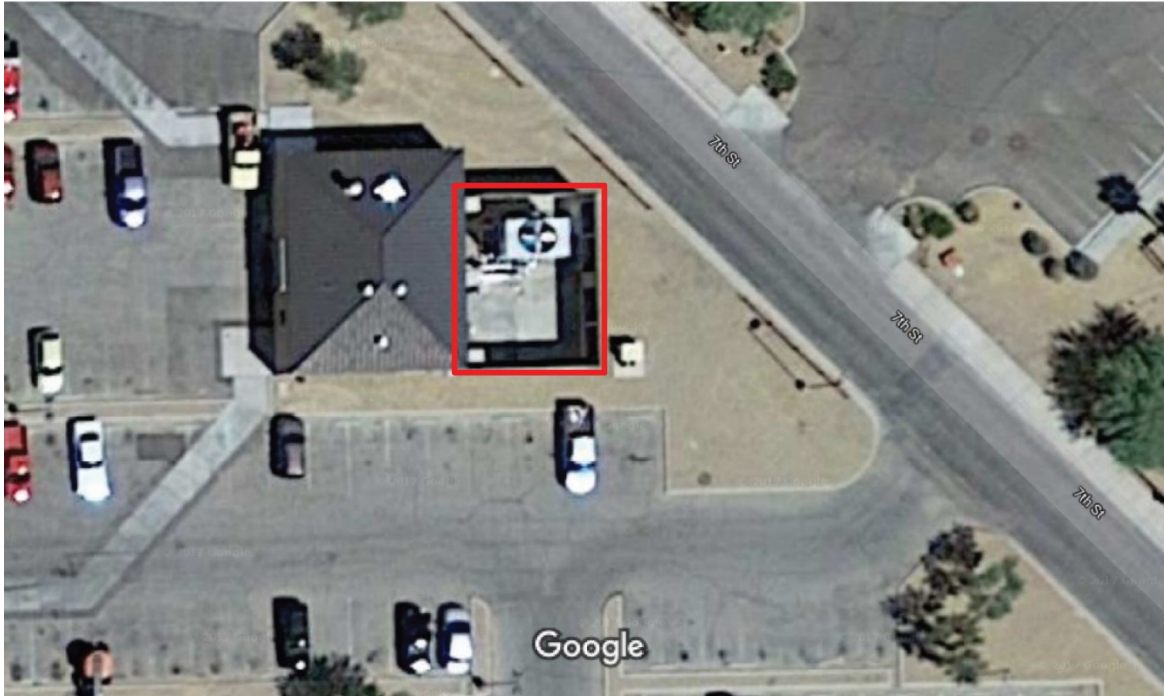
Figure 3. Satellite view of Fort Irwin Building 263 cooling tower enclosure (courtesy of Google).
