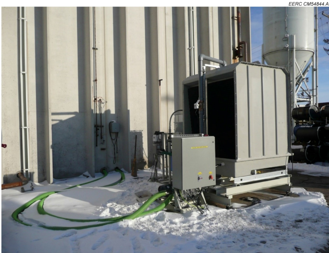
Figure 10. Tower and pump skid with electrical cabinet.
