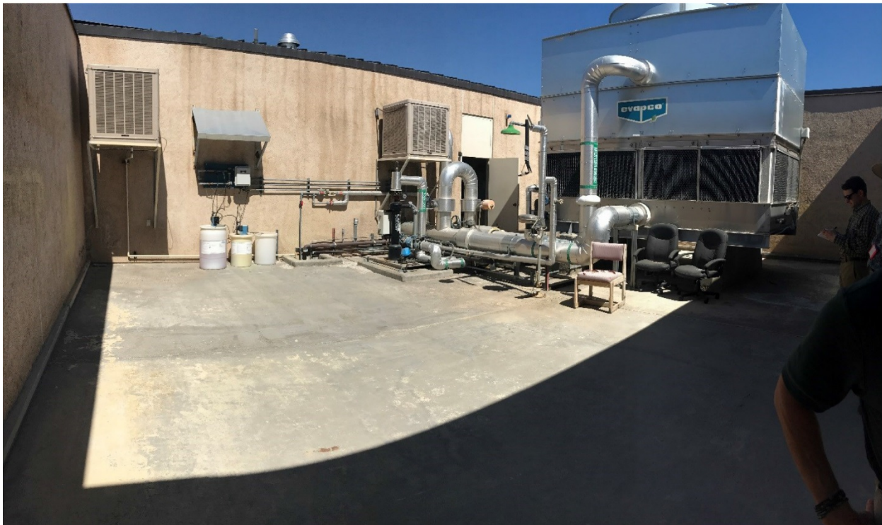
Figure 4. Interior of Fort Irwin Building 263 enclosure.
