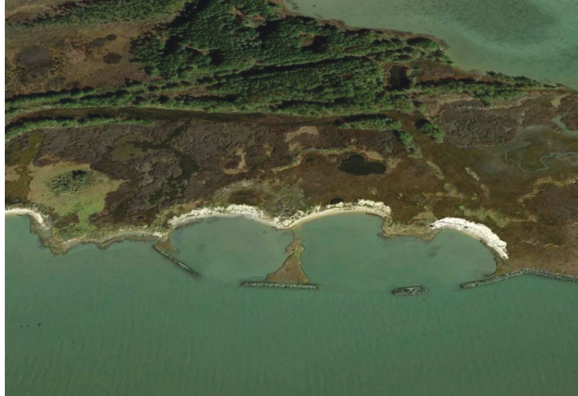
Figure 6. Barren Island segmented breakwaters designed and constructed to promote natural tidal flows to stabilize coastal marsh habitat (Images sourced from Google, DigitalGlobe 2017).
