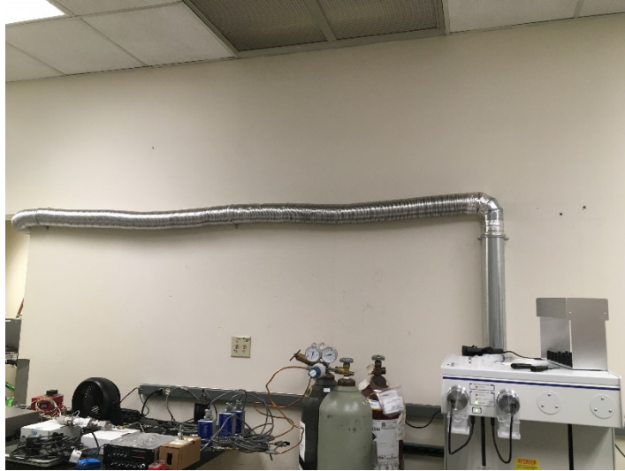
Figure 2. Ventilation duct installed by ASU facilities.
