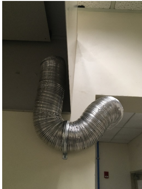
3. The ventilation connects the instrument to a venting hood.
