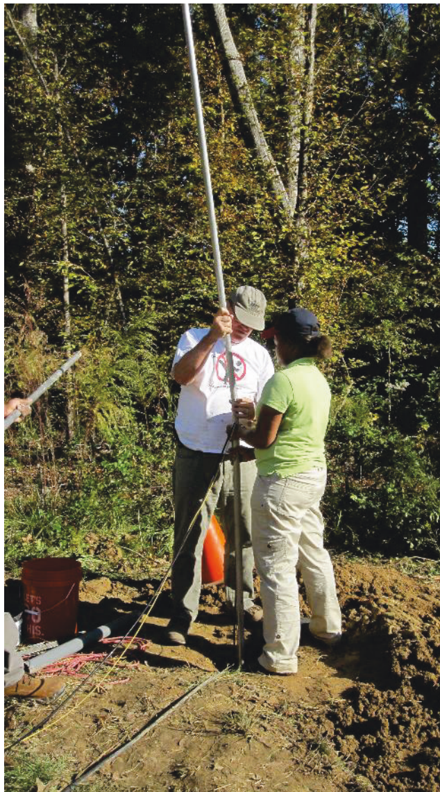
Figure 11. Adding segments to the installation tool.
