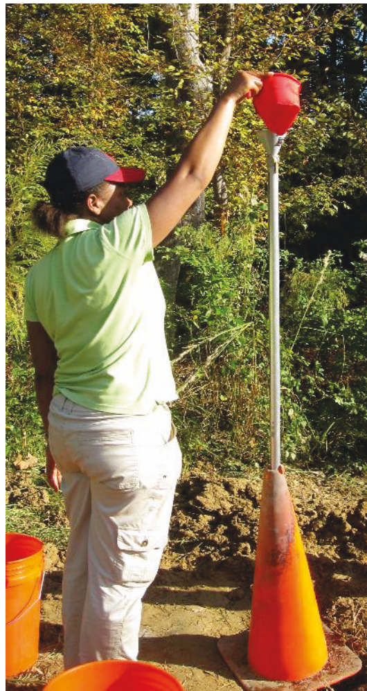
Figure 16. Pouring water into top of install tool for cementing sensor coupling.
