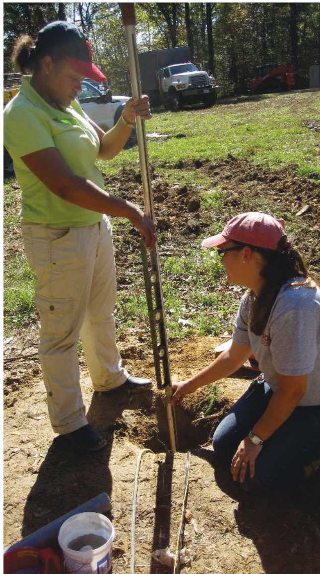
Figure 12. Levelling sensor using install tool and 3-way bubble level.
