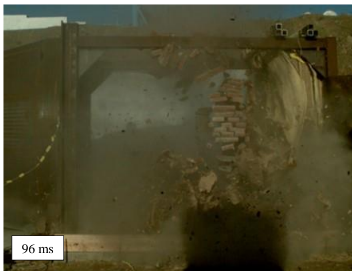
Figure 13. Later-time failure of the brick wall in Test 40 as recorded by the overview HSV camera.
