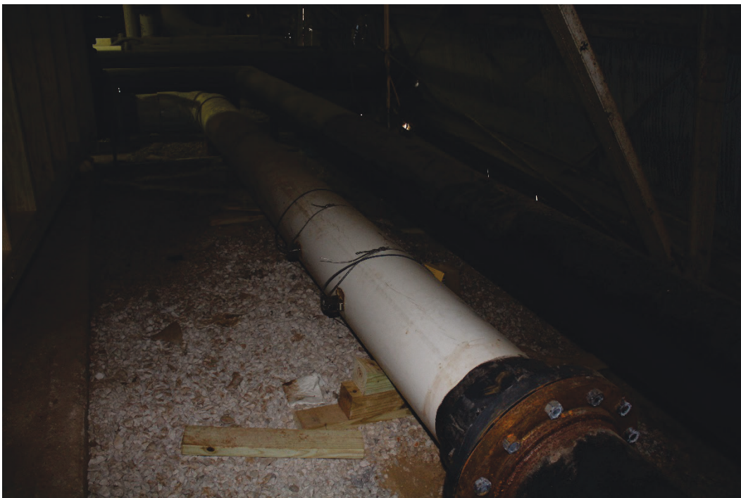
Figure 15. Ultrasonic flowmeter sensors location.
