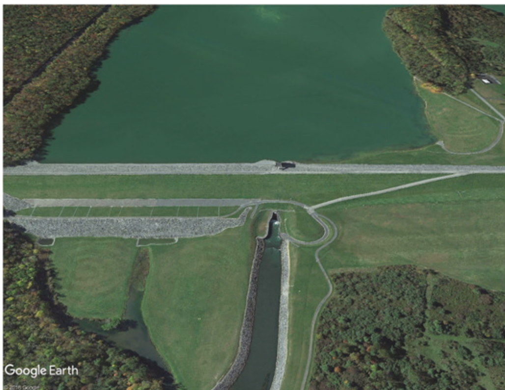
Figure 1. Photograph of Foster Joseph Sayers Dam and Outlet Works (Google Earth).
