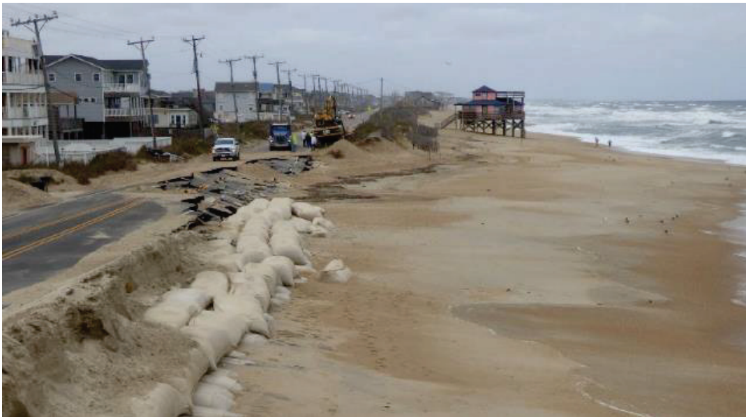
Figure 9. Damages resulting from an overtopped beach berm in Kitty Hawk, NC.
