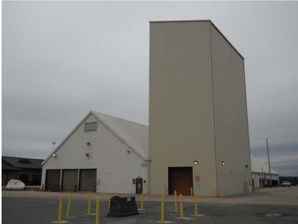
The newly constructed parachute tower for the Lockheed C-130J Super Hercules mission stands complete as an addition to the existing building 259. (Photo taken by Mr. Benjamin D. Herrington, 314 AW/HO; USAF Photo). 84
