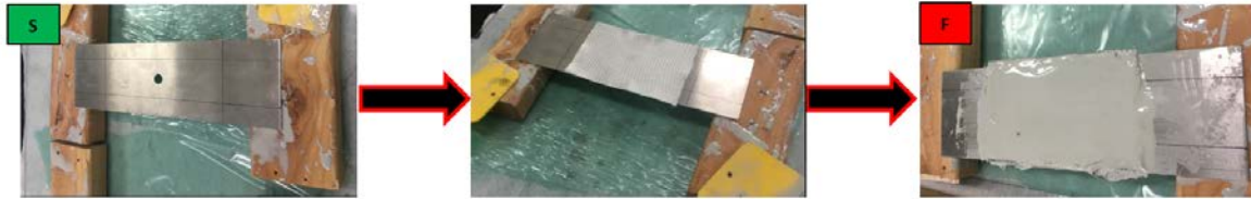
Figure 64. Dry Patching Process Photos
