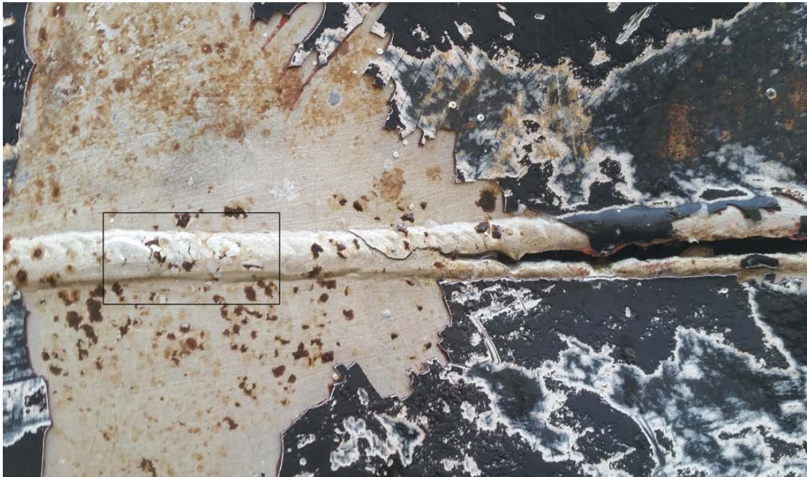
Figure 2. USS Coronado Underwater Cracks: Vertical and Horizontal along Weld Seam. Source: [4].
