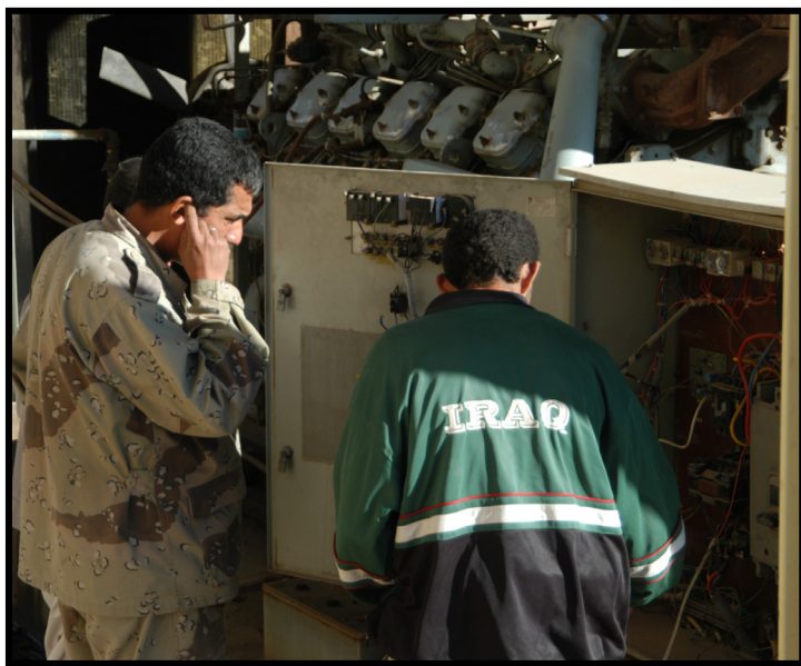
Iraqi municipal workers try to fix a generator in sewer water lift station during Operation AL FAJR (Nov 04)
