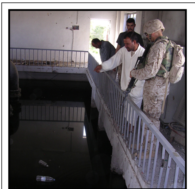
Civil Affairs inspects repairs on pump house outside Fallujah (Sep 04)
