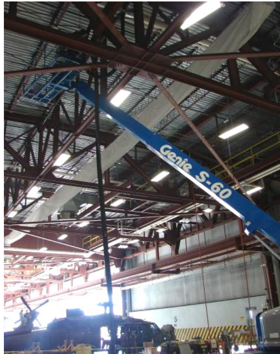
Figure 4. Manlifts were used to reach the connections near the ceiling.
