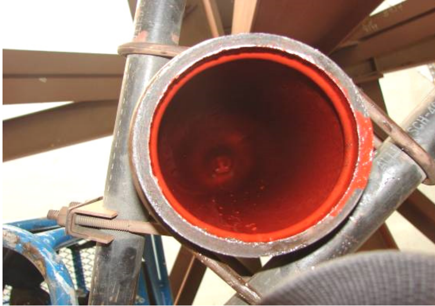
Figure 6. Inside the deluge system's main pipe after epoxy lining.
