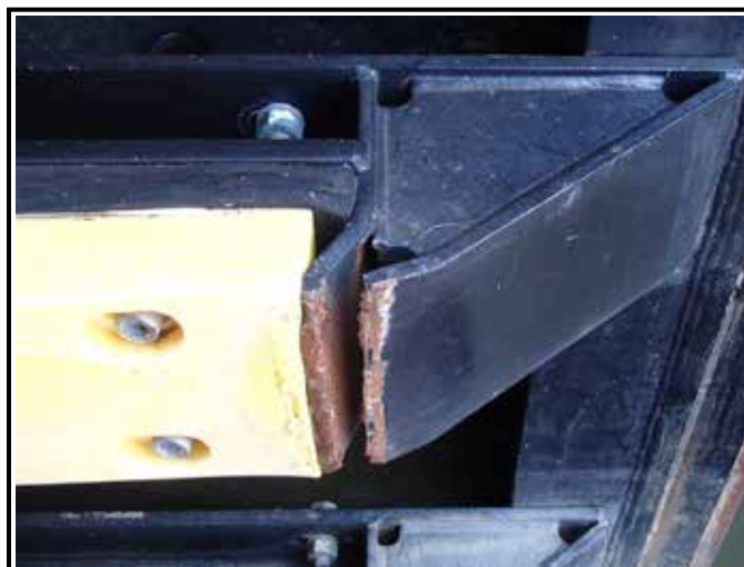
Figure 2-19. View of typical plate deformation and broken weld at the fender guard transition (Greenup L&D).
