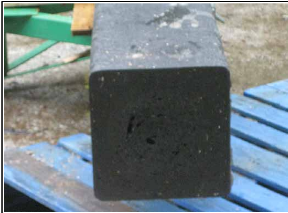
Figure A-12. HDPE timber with typical void formations in the center core.
