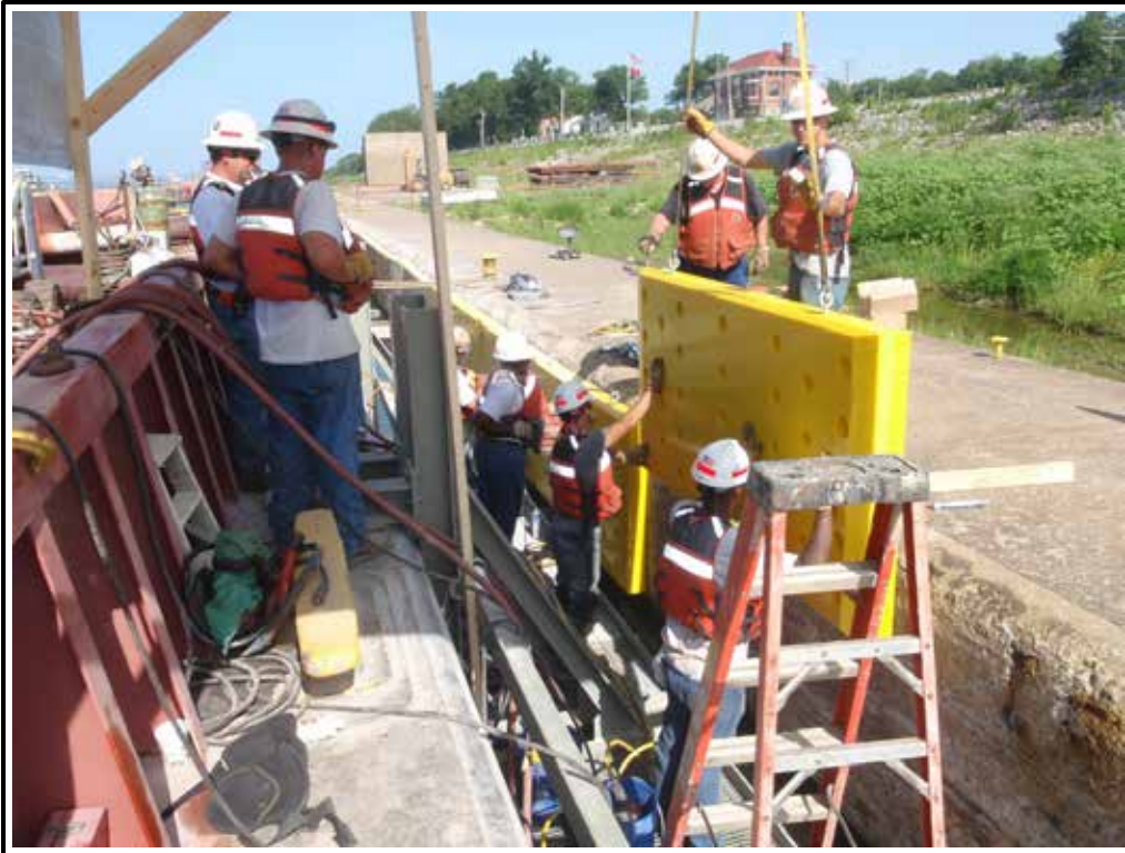
Figure A-11. UHMWPE panel on deteriorated armor wall (Ohio River Lock #52).
