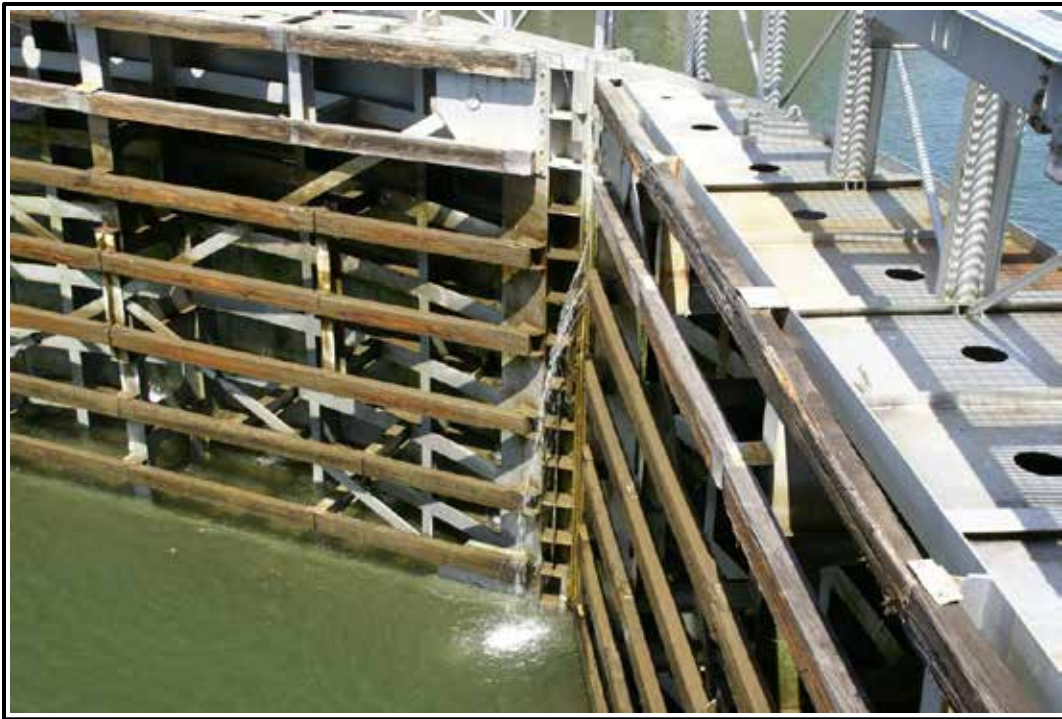
Figure 2-1. Typical wooden fender installation.
