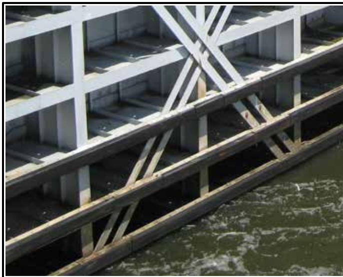
Figure 2-18. Fenders at Lockport Lock and Dam, Lockport, IL.
