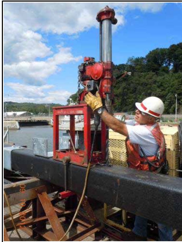
Figure 2-21. Pre-drilling the attachment points.
