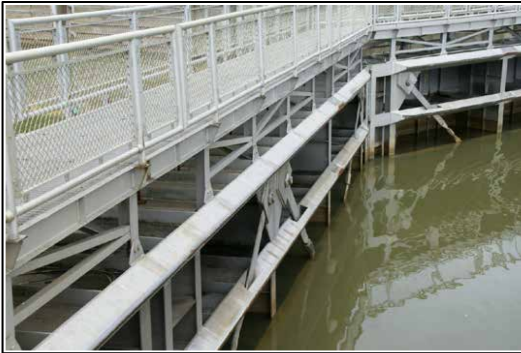
Figure 2-3. Triangular steel fenders.
