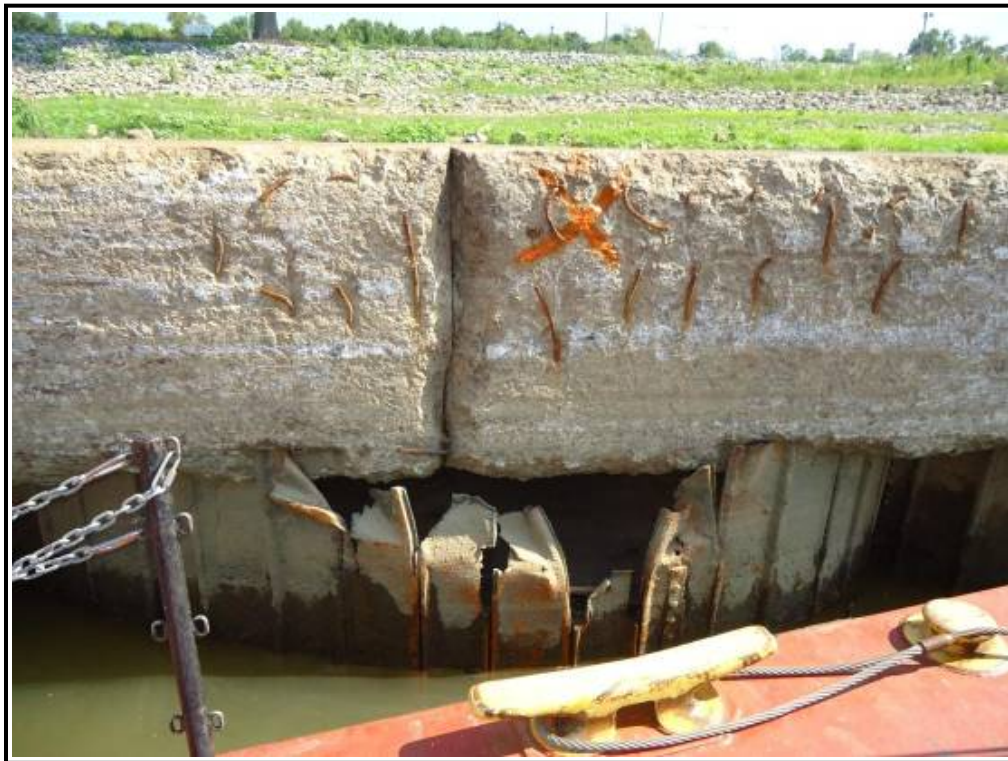
Figure A-10. Deteriorated wall due to barge rubbing (Ohio River Lock #52).
