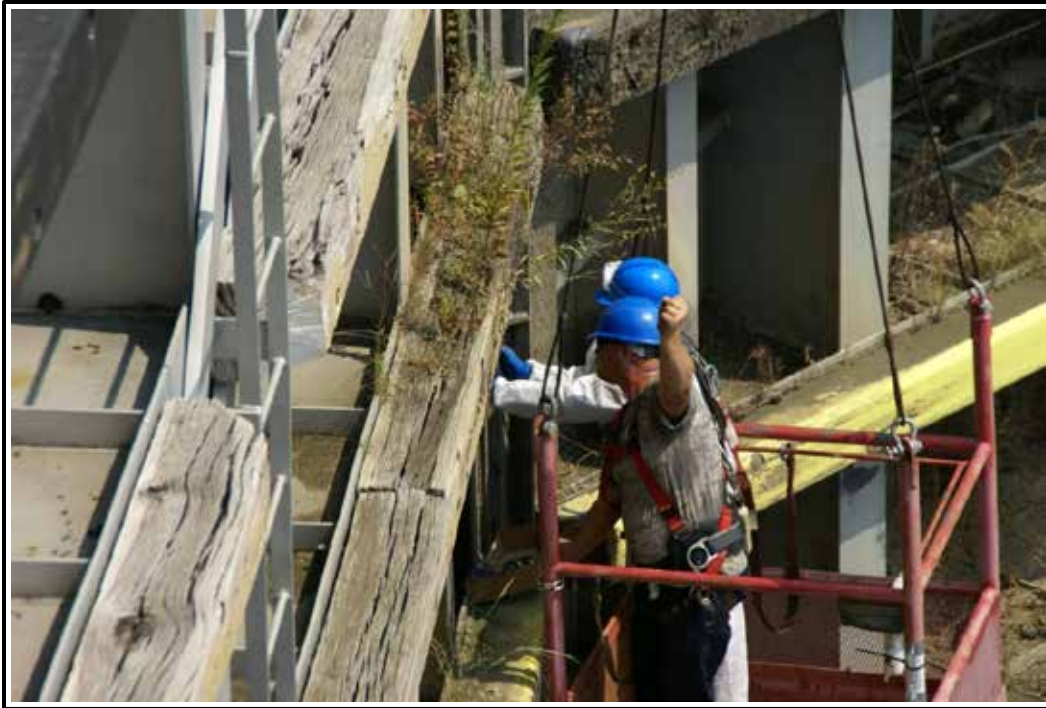
Figure A-3. Fender repairs. Notice vegetation growing out of the timber.
