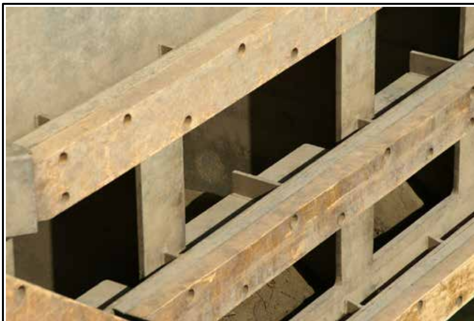
Figure 2-6. Layered UHMWPE and elastomeric fenders (Olmsted L&D).
