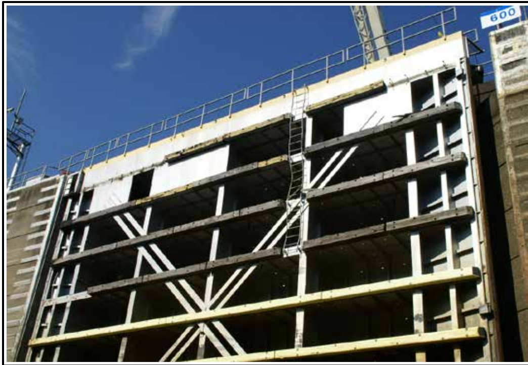
Figure A-5. Various fender types and damaged ladder.
