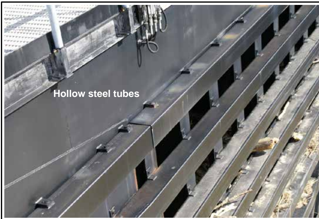
Figure 2-4. Square tubular steel fenders (Winfield L&D).
