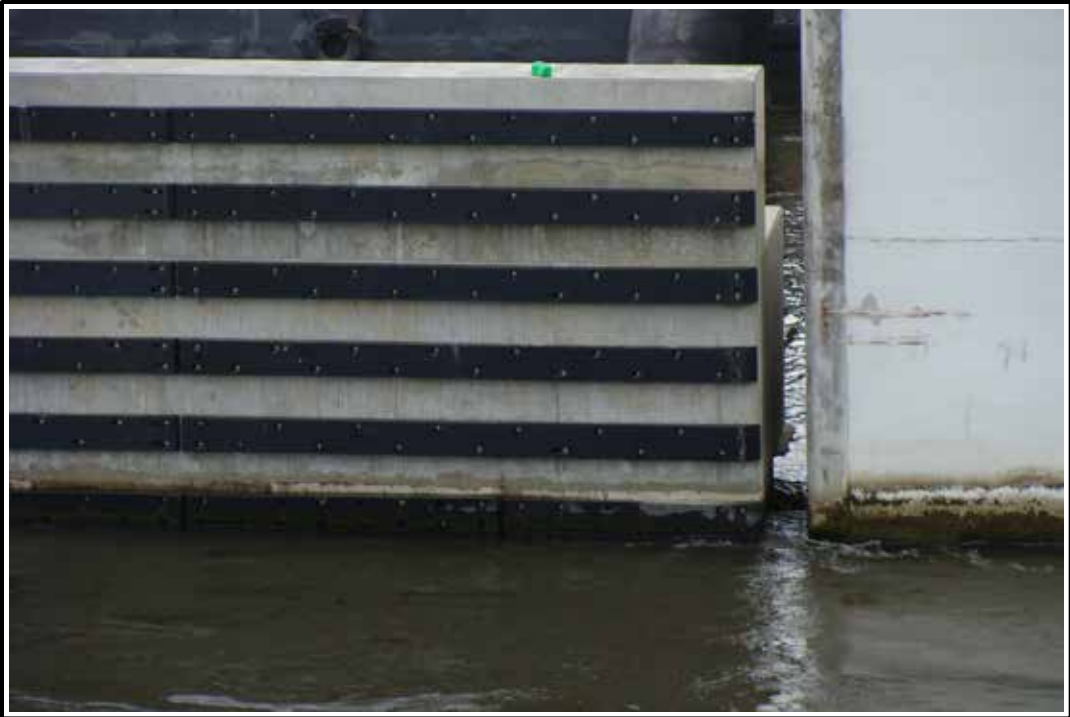
Figure A-7. Approach wall with HDPE fenders (Lake Borgne Surge Barrier).
