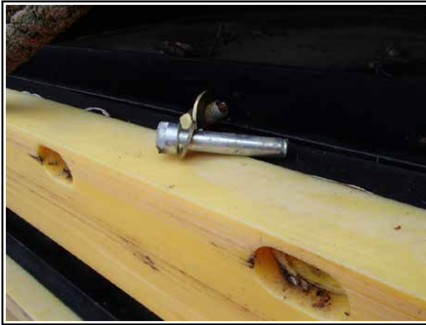
Figure B-2. Greenup Lock and Dam, main chamber upstream river wall leaf, view of sheared off machine bolt. Most bolts are bent or sheared off, but stayed in place.
