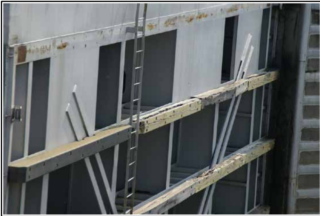
Figure 2-14. Deteriorated wood fenders and one replacement HDPE fender.
