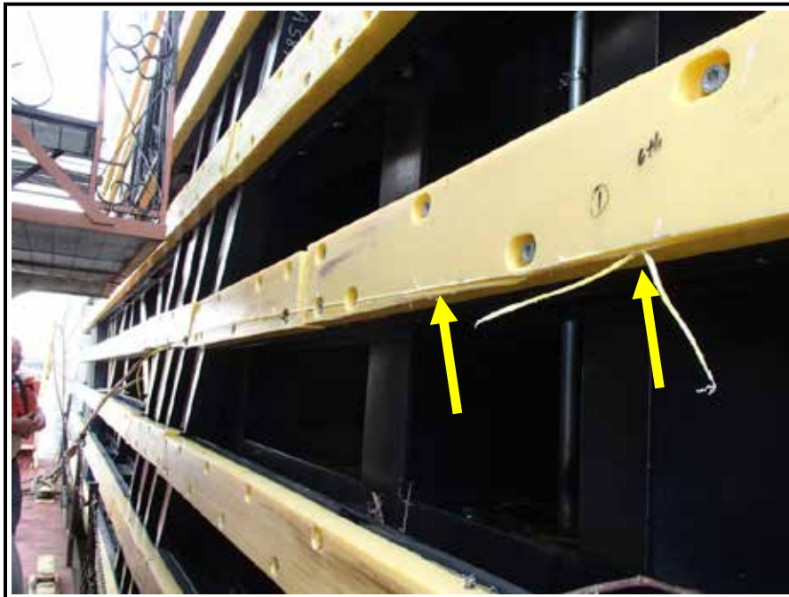
Figure B-3. View of gouges in UHMW fender.
