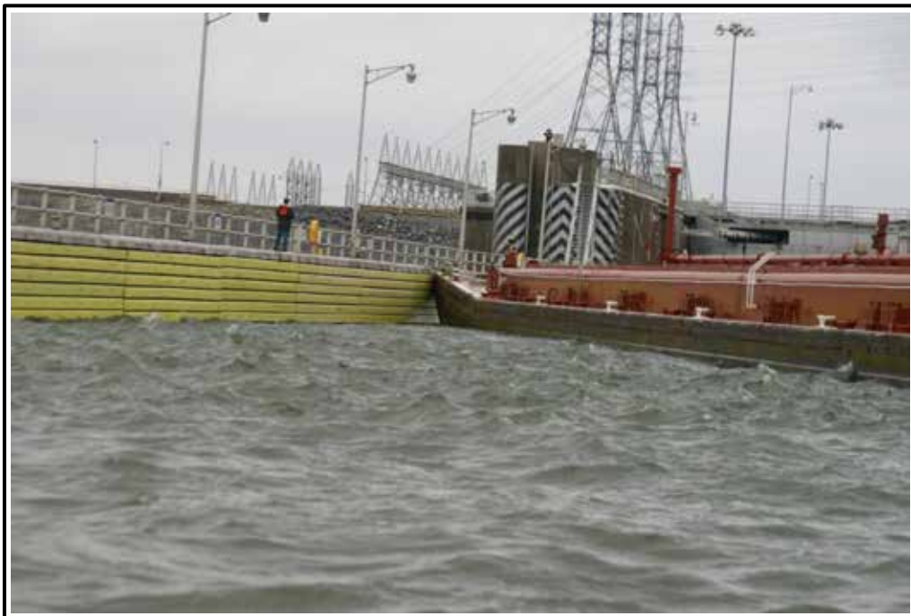
Figure 2-15. Kentucky Lock upstream approach wall with yellow fenders for better visibility.
