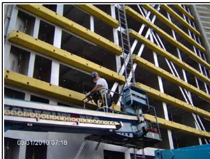
Figure A-2. Installation of HDPE fenders colored yellow for visibility.
