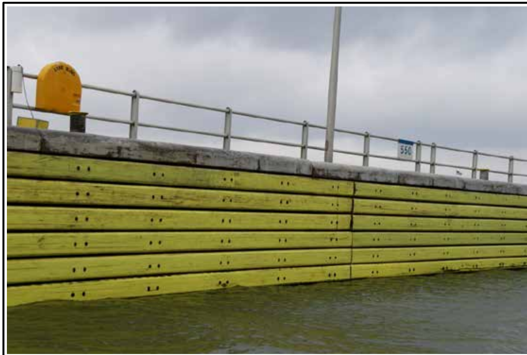
Figure A-6. Approach wall with yellow HDPE fenders (Kentucky Lock).
