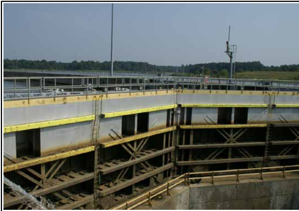
Figure A-4. Various fender types and damaged ladders.
