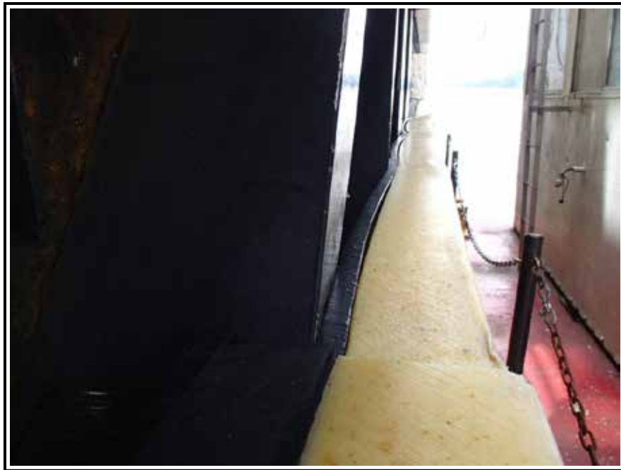
Figure B-4. Greenup Lock and Dam, main chamber upstream river wall leaf, view of bent protection plate over the diagonals.
