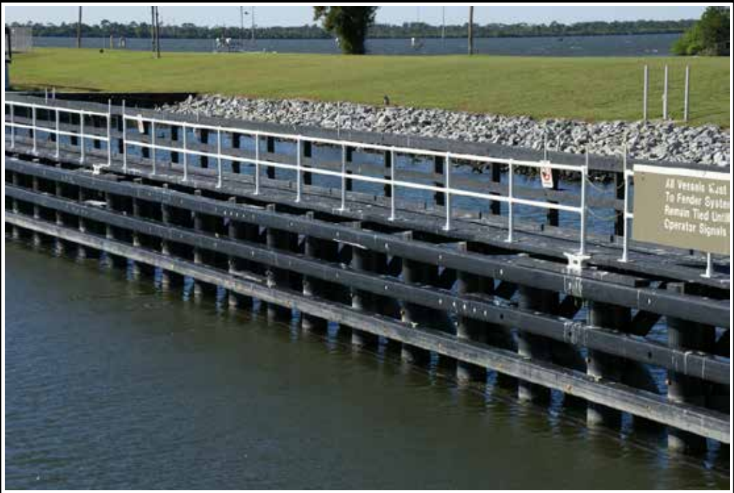
Figure A-8. Guidewall with HDPE fenders (Port Canaveral Locks).
