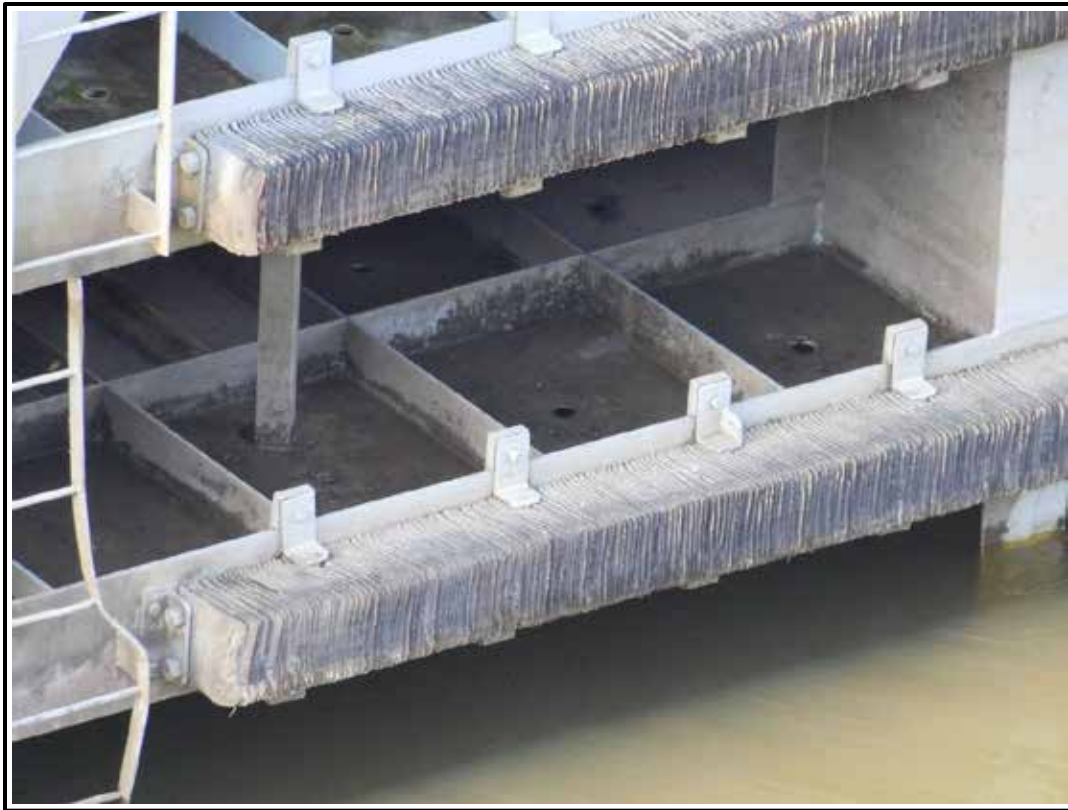
Figure 2-9. Recycled rubber fenders (Holt L&D).
