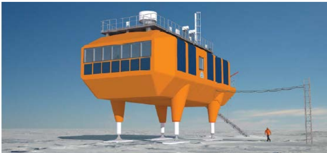
Figure 1. A three-dimensional (3-D) rendering of the planned AWO building installed at Summit Station (AECOM 2012). Four telescoping legs support the building through a lower, structural space frame. The building could be preassembled to include upper frame and exterior insulated panels prior to GrIT transport.
