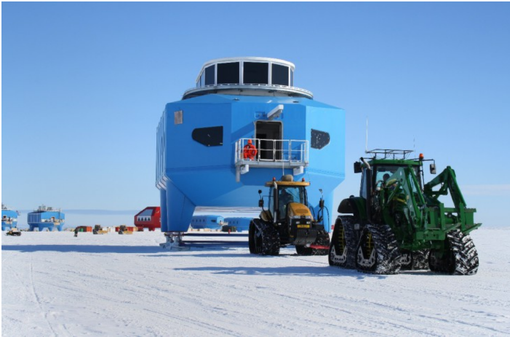
Figure 2. Halley VI modules being towed into place at the Halley Research Station of the British Antarctic Survey. These modules are structurally similar to the proposed AWO building and were designed to be towed on the skis attached to their telescoping legs.
