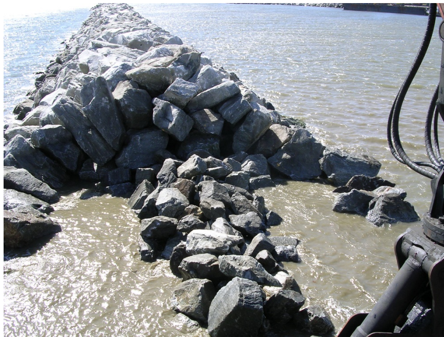
Figure 34. Special stone placement for a breakwater structure.
