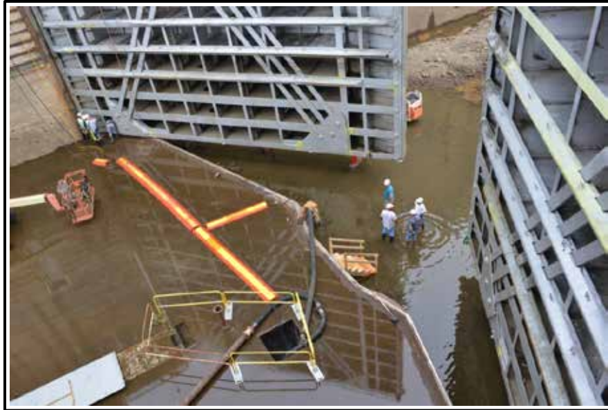
Figure 5. Maintenance worker inspecting a miter gate with the chamber dewatered.
