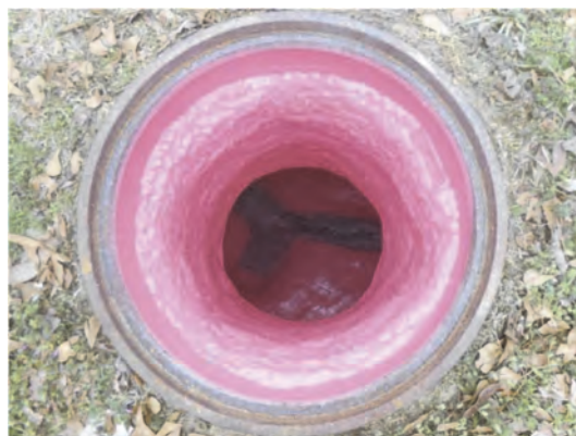
Finished (coated) manhole.
