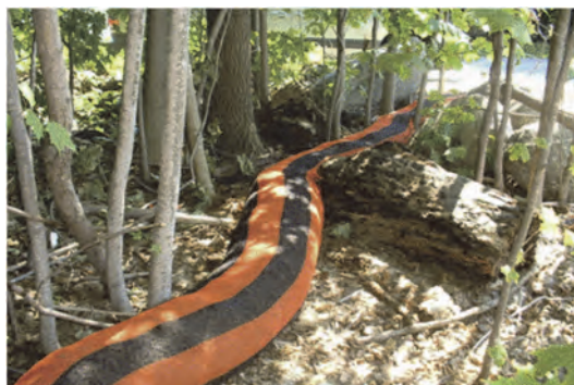
Erosion control filter sock in use under field conditions.
