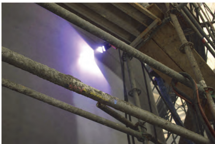
Thermal arc spray application of 85/15 alloy.
