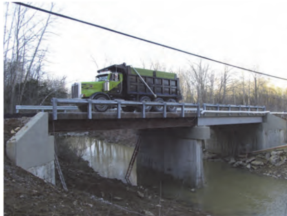
Round 1 Tests: Truck 1 crossing bridge along Path Y3.
