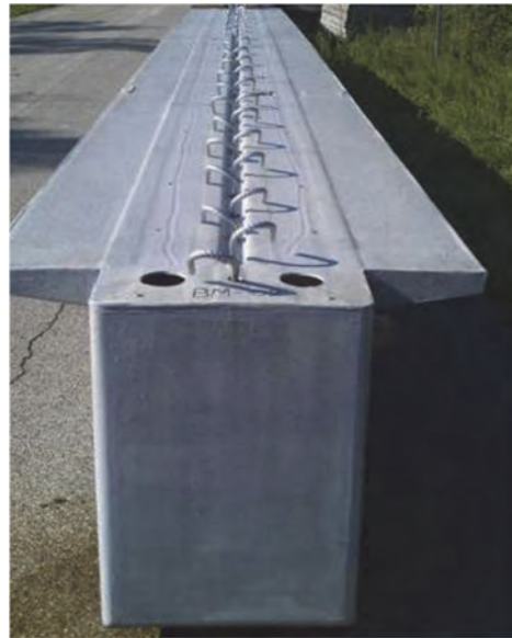
Ports for injecting self-consolidating concrete .
