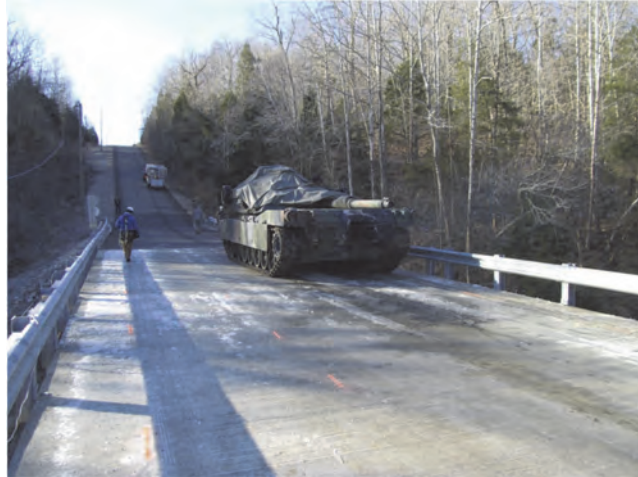
Tank crossing Bridge No. 4, Fort Knox, KY.
