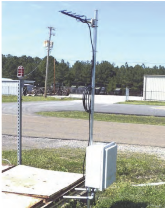
Yagi antenna used for SCADA communications.
