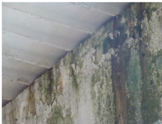
Mold in Fort Polk pumphouse with concrete block walls.
