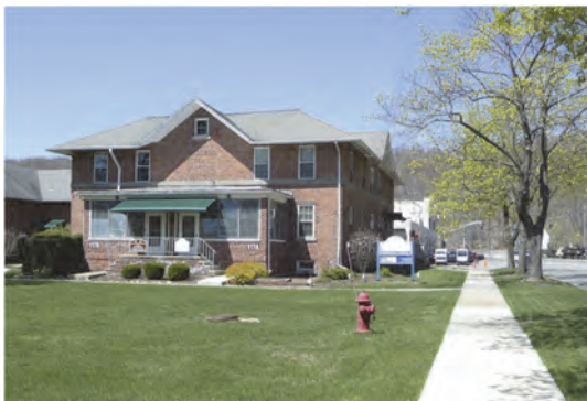
Bldg.117, former stables.
