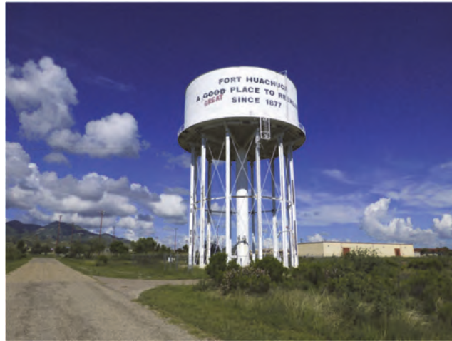
Fort Huachuca, AZ, elevated water tank.
