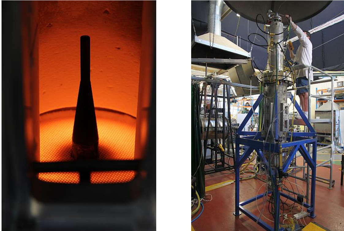
Figure 19: Pressurised burner commissioning.
