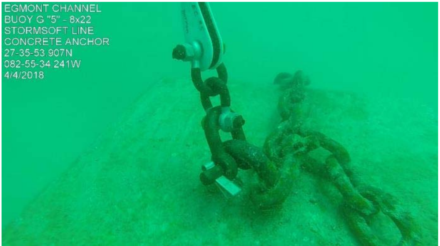
Figure 40. Egmont Channel G "5" StormSoft EFBMS connection to concrete sinker.
