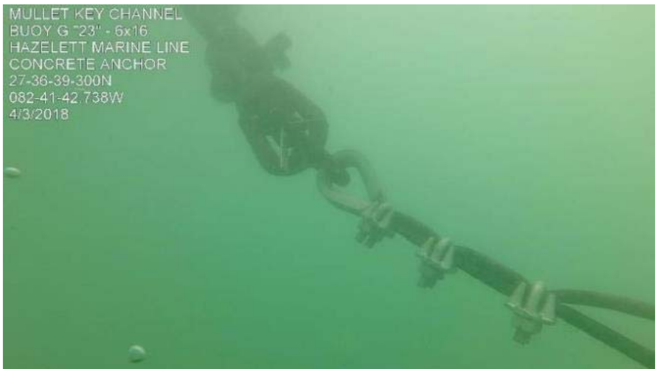
Figure 35. Hazelett Marine EFBMS Uniline connection to CG 3rd Class swivel at buoy bridle.
