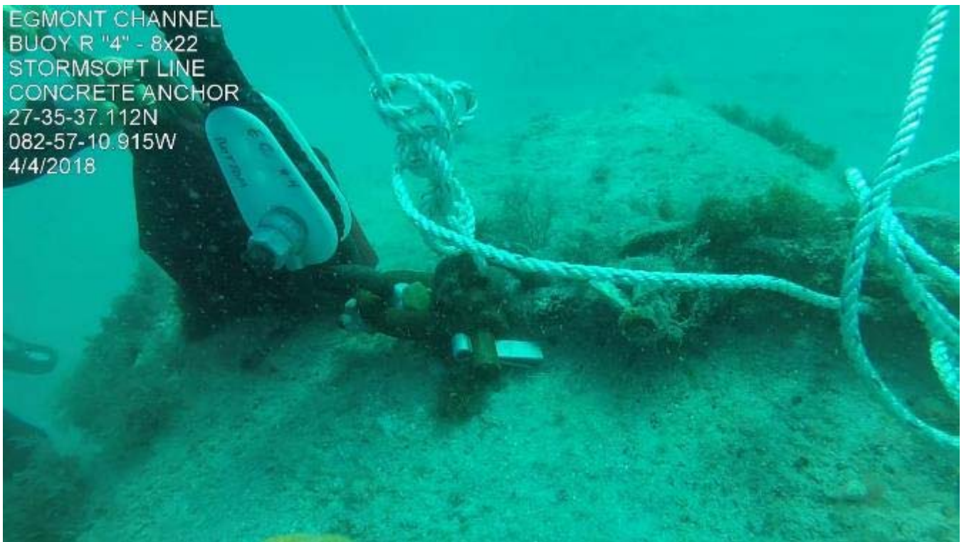
Figure 37. Egmont Channel R "4" StormSoft EFBMS connection to concrete sinker (diver tagline present).
