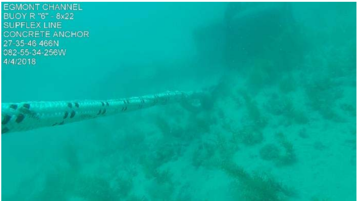
Figure 46. Superflex EFBMS chain/mooring line connection on bottom.
