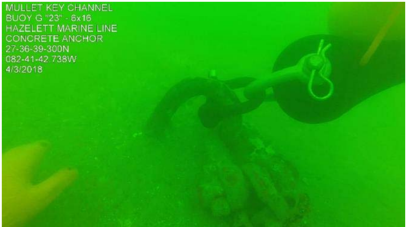
Figure 34. Mullet Key Channel G "23" Hazelett Marine EFBMS connection to concrete sinker.
