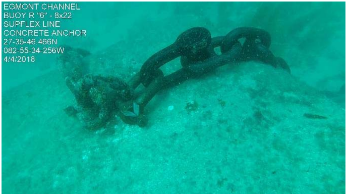
Figure 43. Egmont Channel R "6" Superflex EFBMS connection to concrete sinker.
