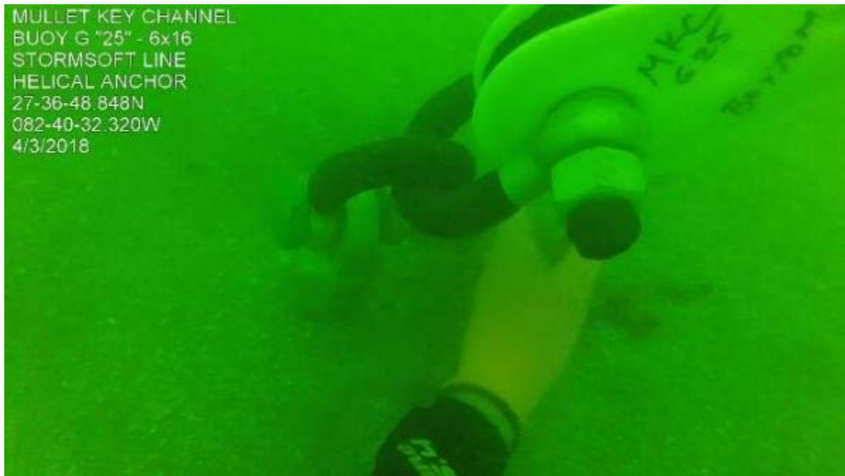
Figure 32. Mullet Key Channel G “25” helix mooring termination head with StormSoft EFBMS.
