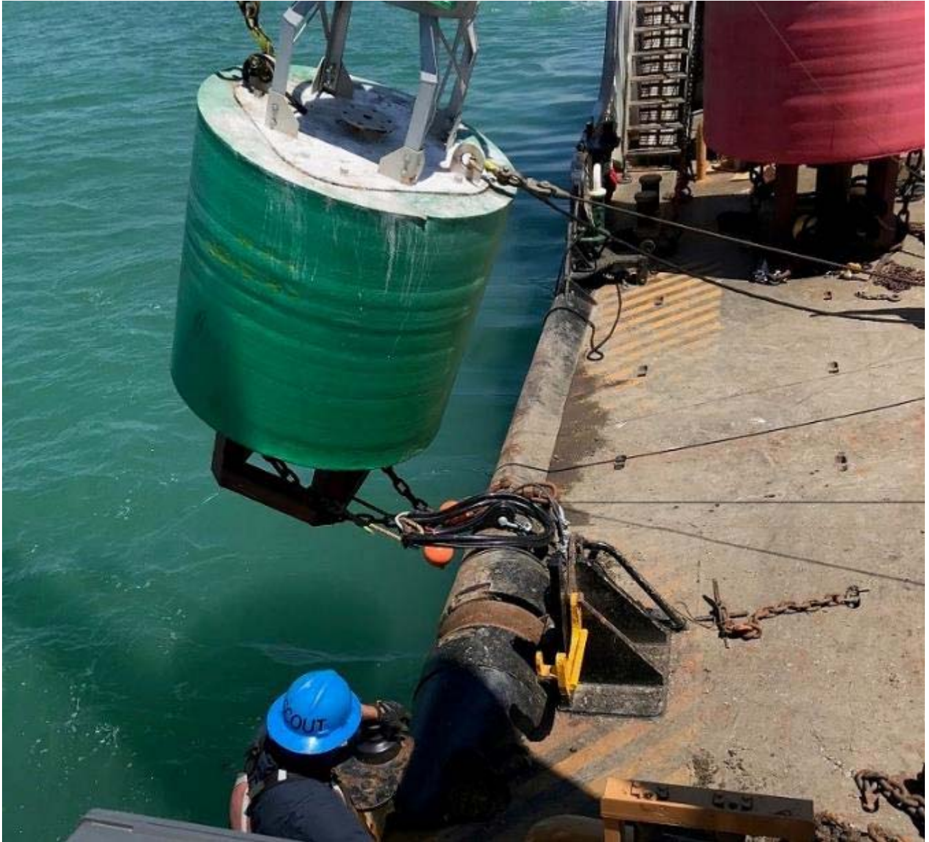
Figure 33. RDC-provided 6X16LFR buoy with Hazelett Marine mooring.
