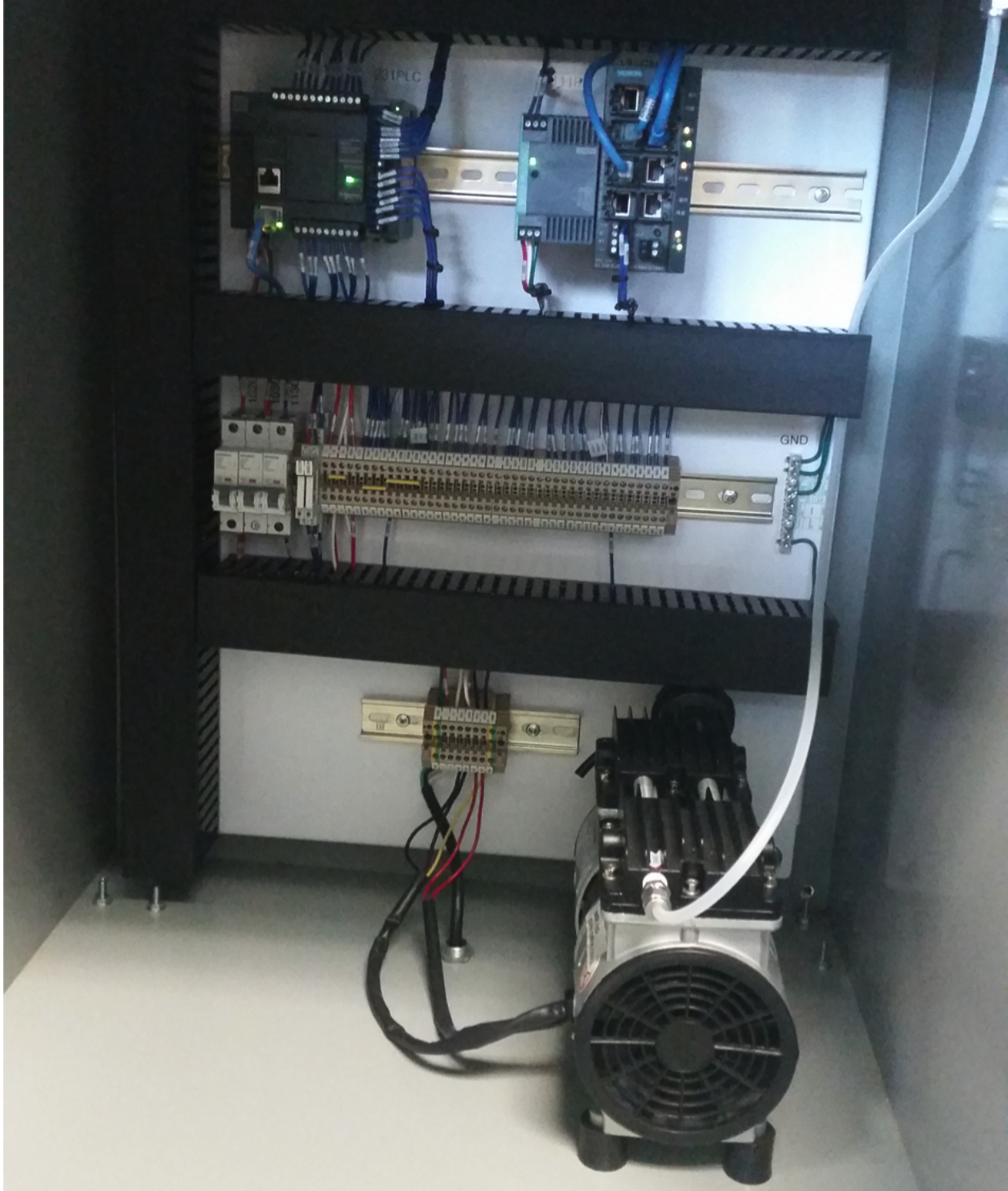
Figure 3: Cabinet-view of the gas pipeline simulator
