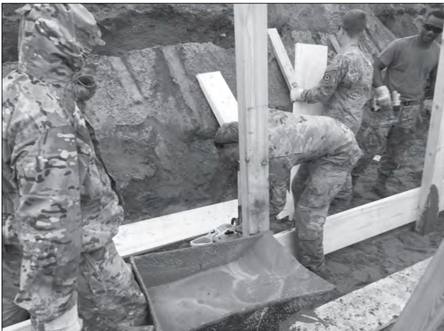
Soldiers construct a trench.
