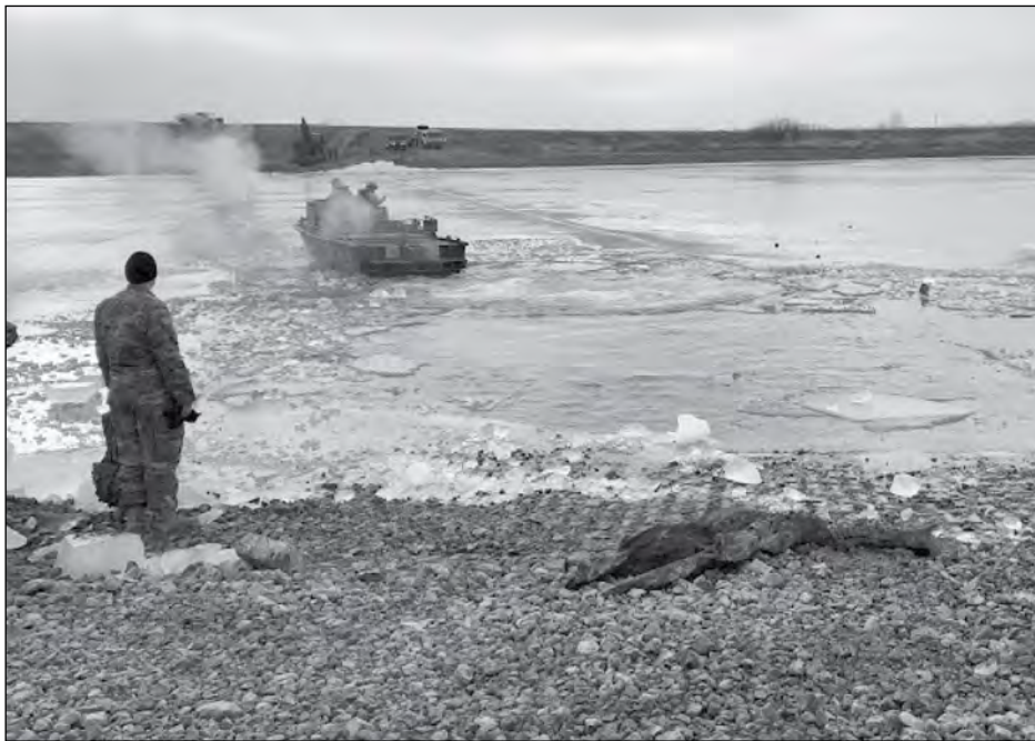
BEBs and an excavator were used to break and clear large chunks of ice from the channel.
