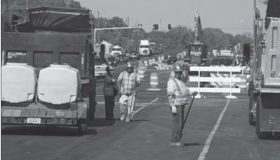
Asphalt trucks line up to place asphalt along Vint Hill Road, Manassas, Virginia. A key part of asphalt placement is traffic management, as roads are built under normal operational traffic conditions.
