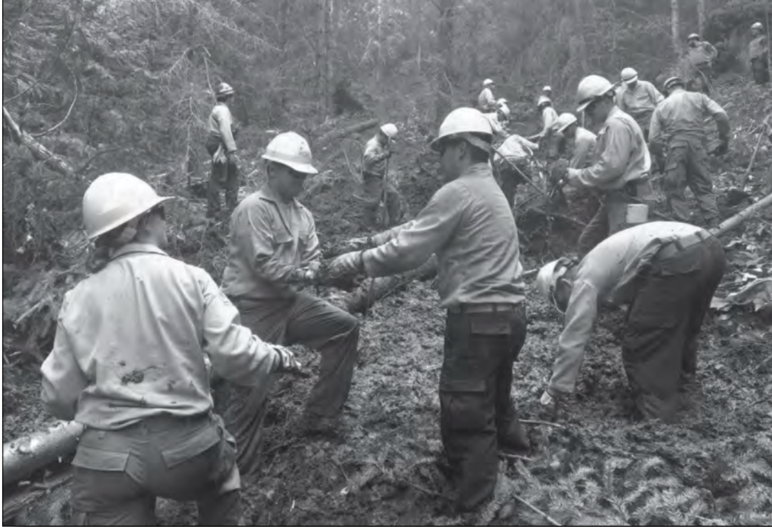
Soldiers install interceptor dikes.
