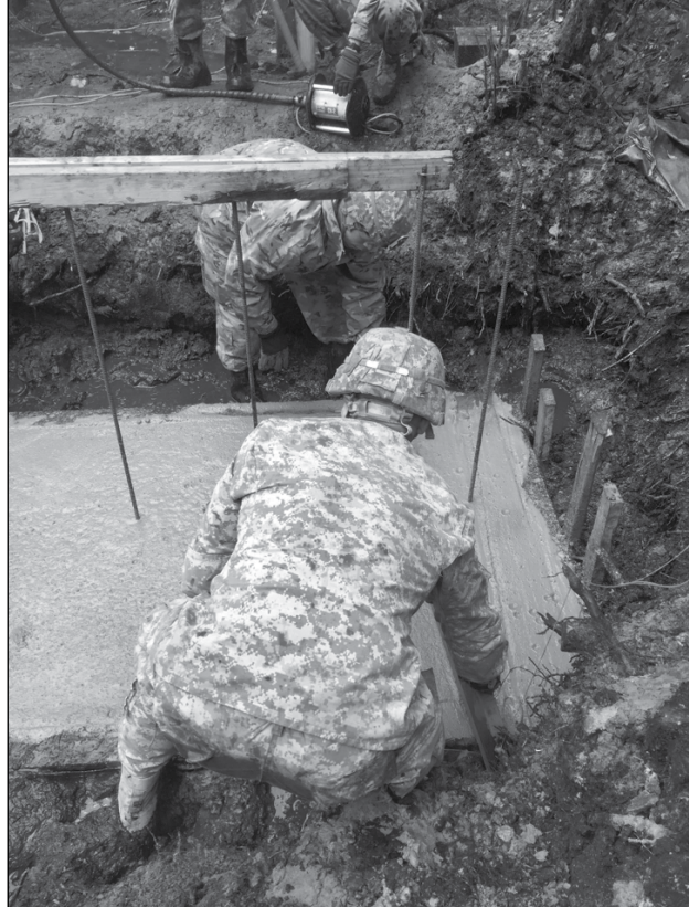
3d Platoon emplaces formwork and rebar for a vertical-construction concrete pour.
