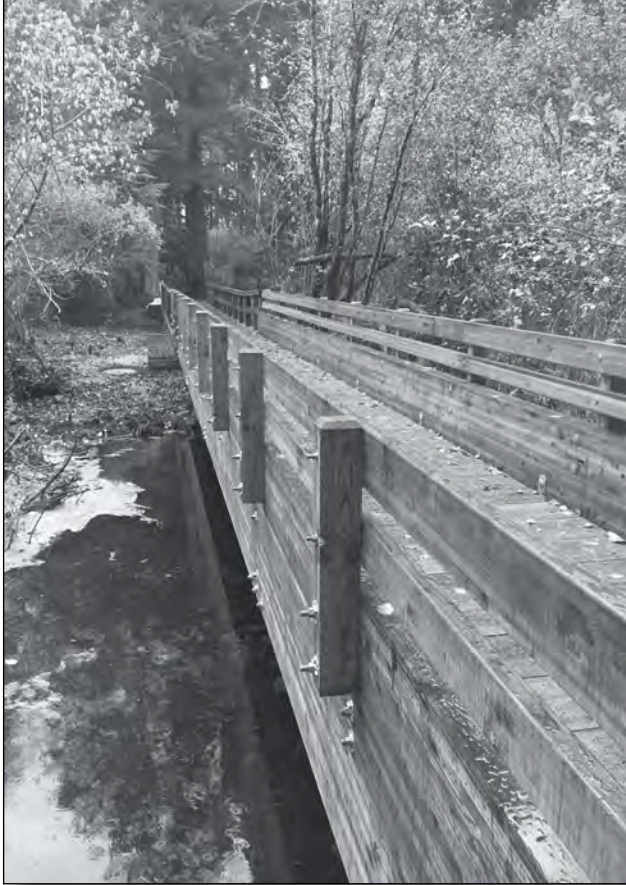
The fully assembled bridge across Murray Creek
