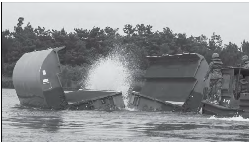
Bridge crew members assembling an improved ribbon bridge.
