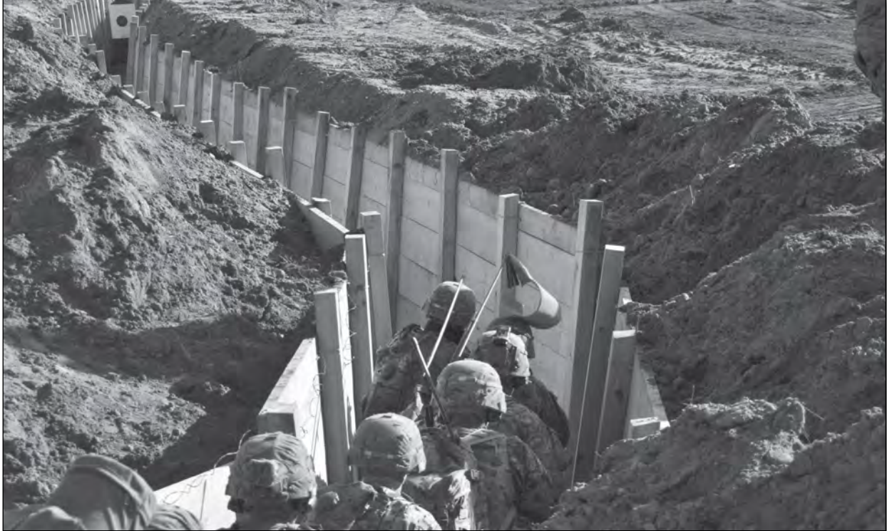
Soldiers from the Engineer Squadron, 2d Cavalry Regiment, built a trench to create a realistic training environment for a troop size element.
