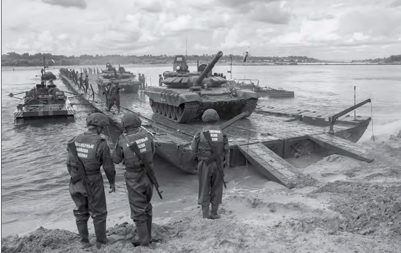
Pontoon bridging operations
