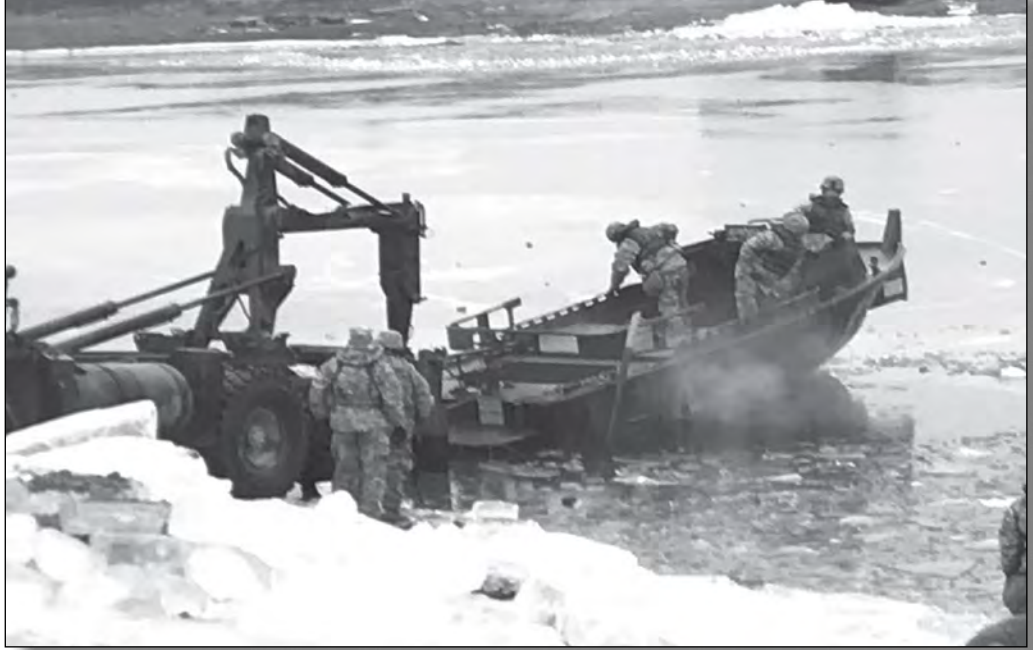
Members of the 143th attempt to break through the ice on Day 1 using the weight of a bridge erection boat.
