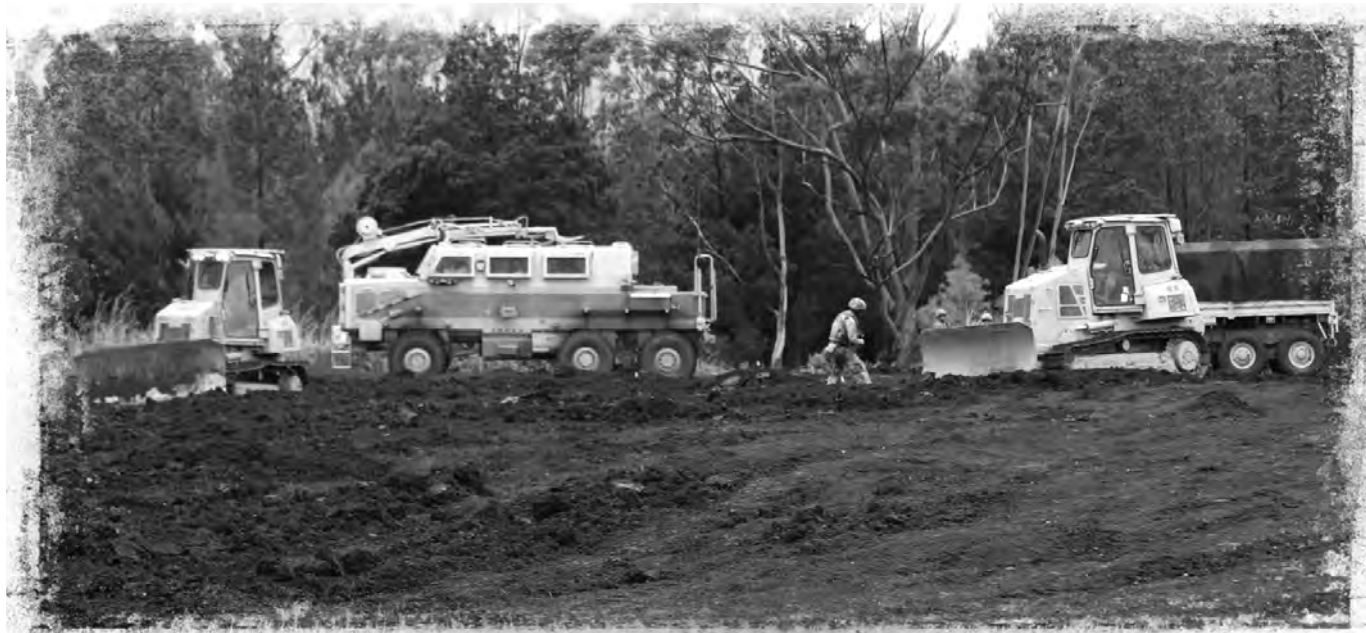
The 95th Clearance Company provides security as the 523d Engineer Company begins emplacing counter-mobility obstacles.
