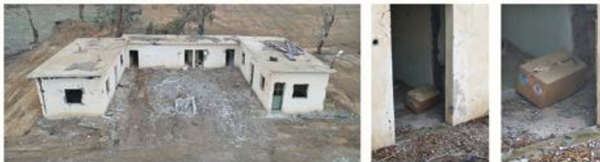
Images from a small unmanned aircraft (SUA) show the extent of structural damage, then close-up views of visible suspicious items.
