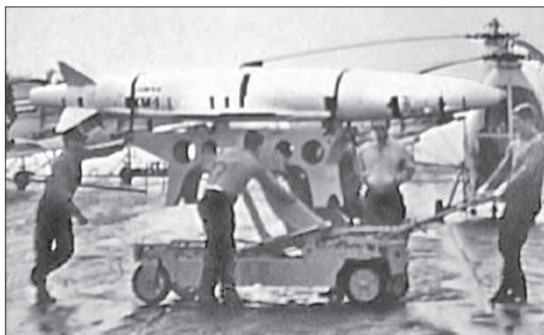
The Naval Ordnance Laboratory's XASM-N-8 Corvus being prepared for test, circa 1958.
