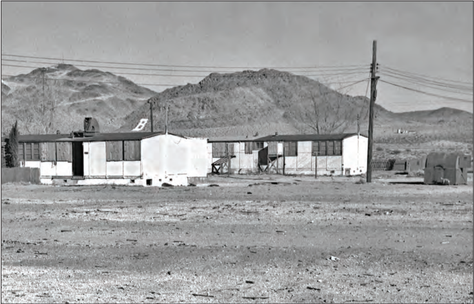
Deteriorating 1940s-era prefabricated housing units off Richmond Road, 1960. B Mountain, complete with painted “B,” is in the background.
