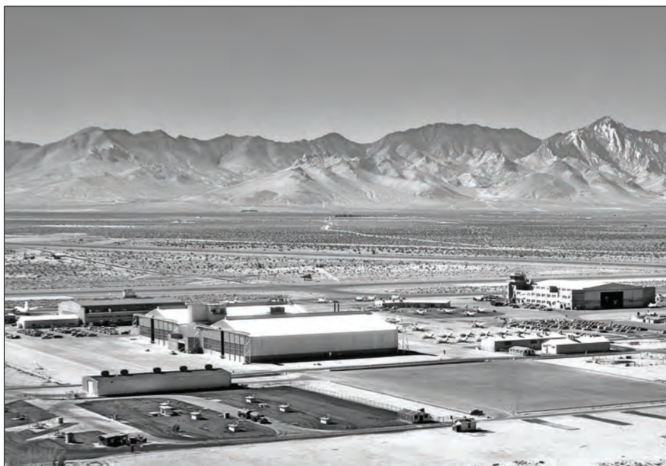
Armitage Field after construction of Hangar 3, the large two-bay building at center left. Hangar 2 is at left, with Hangar 1 at right. The view is west toward the Sierra Nevada.
