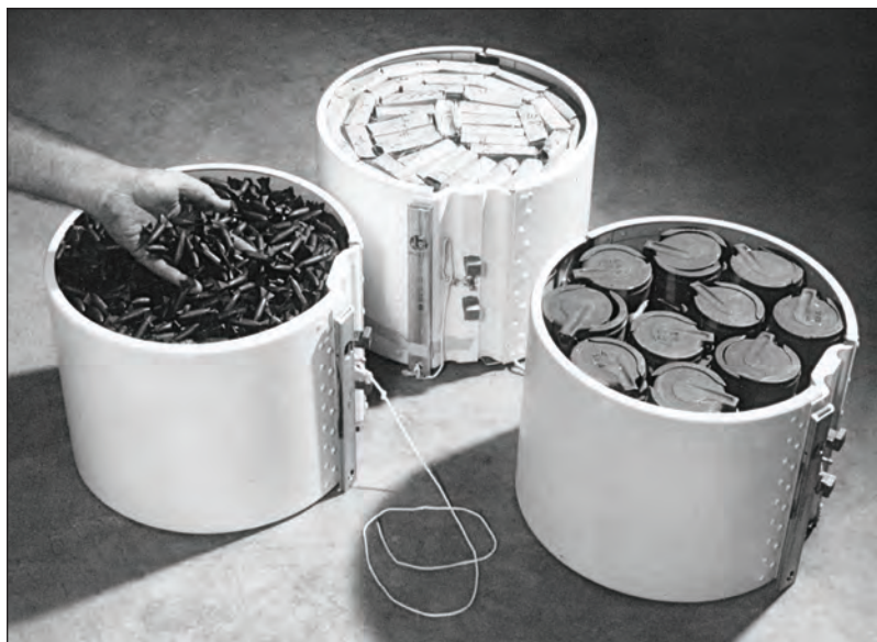
Gladeye canisters loaded with Lazy Dog projectiles, leaflets, and munitions.
