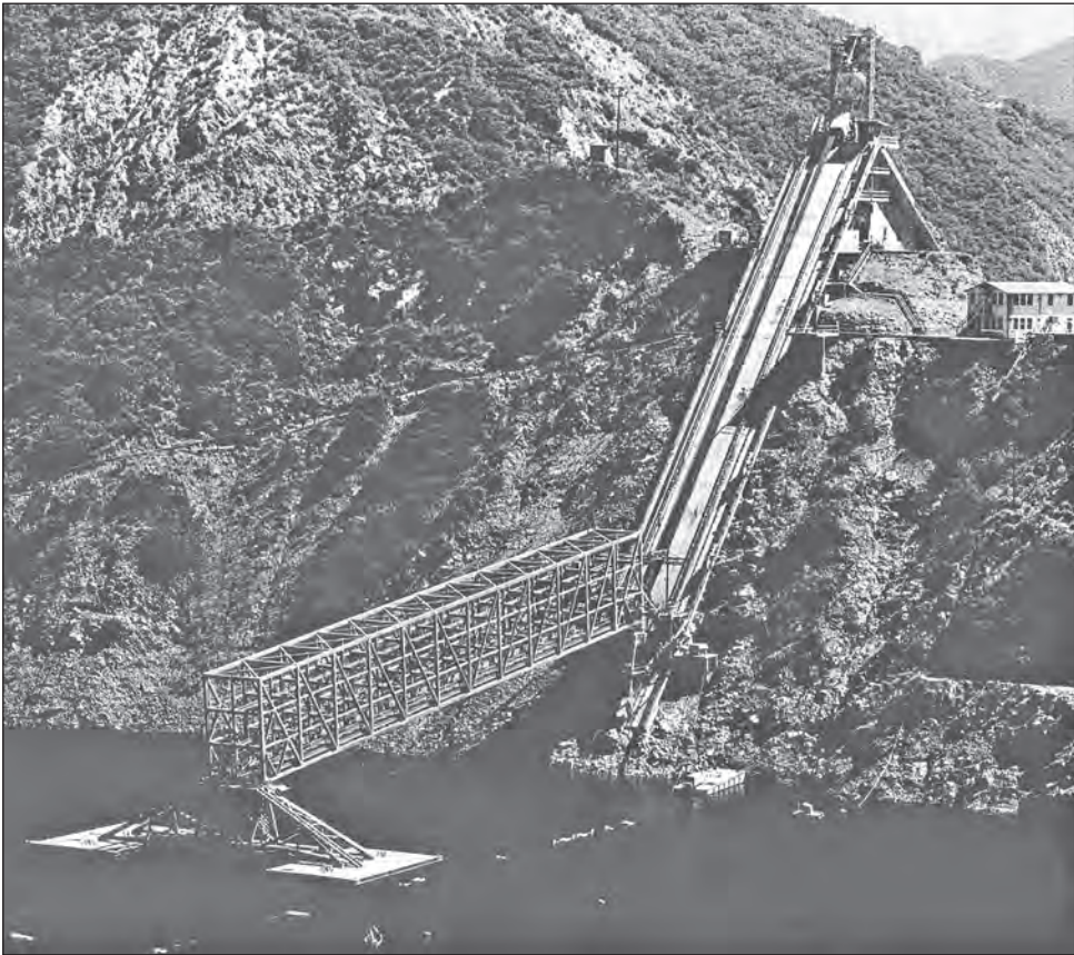
Variable-Angle Launcher at Morris Dam.
