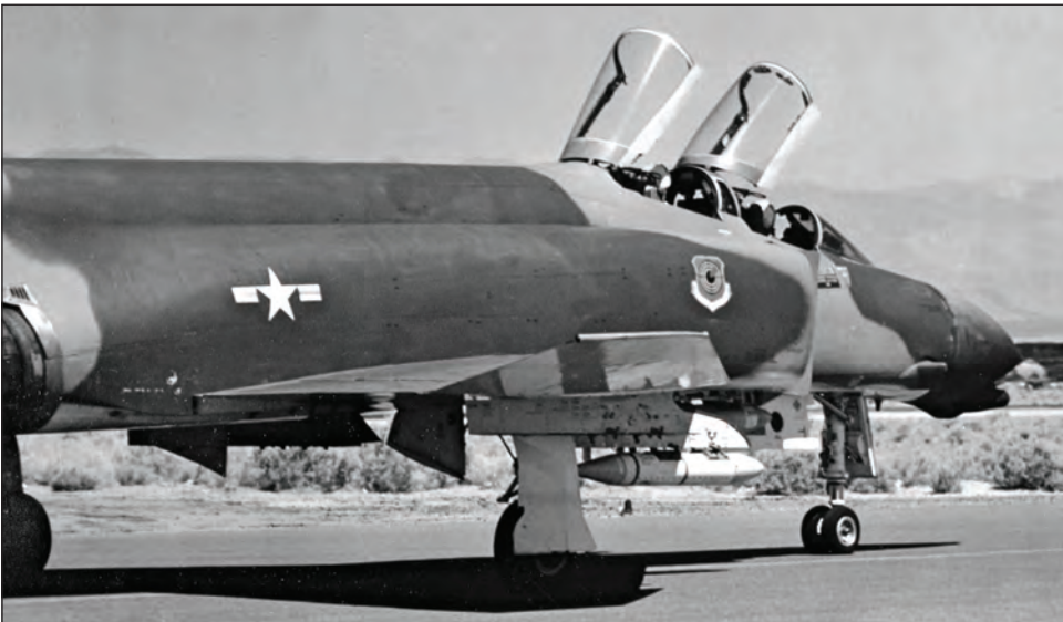
Seek-Bang nuclear Walleye on Air Force F-4 aircraft.
