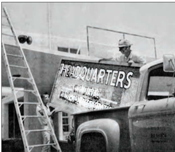
Joe Paiement and Wilbur Beard of Public Works taking down the NOTS sign from the Administration Building, July 1967.
