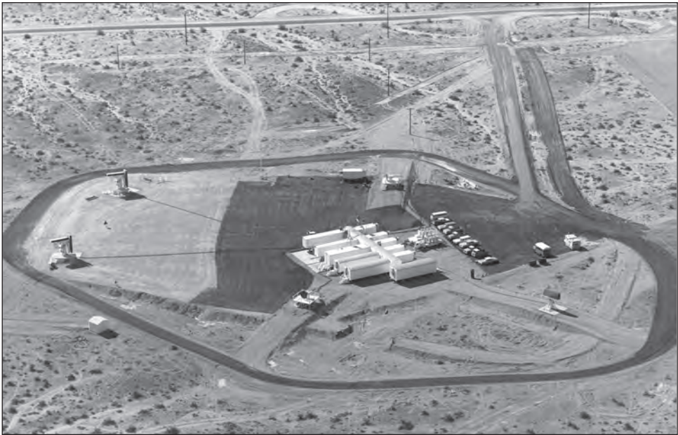
Typical threat radar installation at Echo Range, circa 1968.
