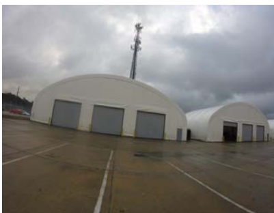
Tension Fabric Shelter
