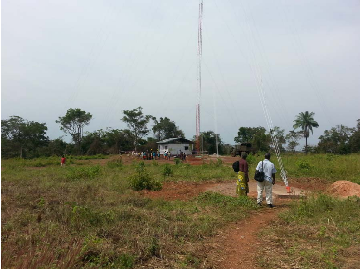
Figure 17. SOCFWD Radio Station Construction in Djemah, CAR.
