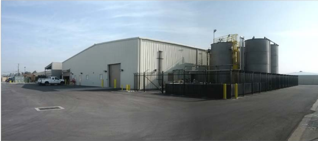
Figure 5.16 Photo of Full-scale Groundwater Treatment Plant.
