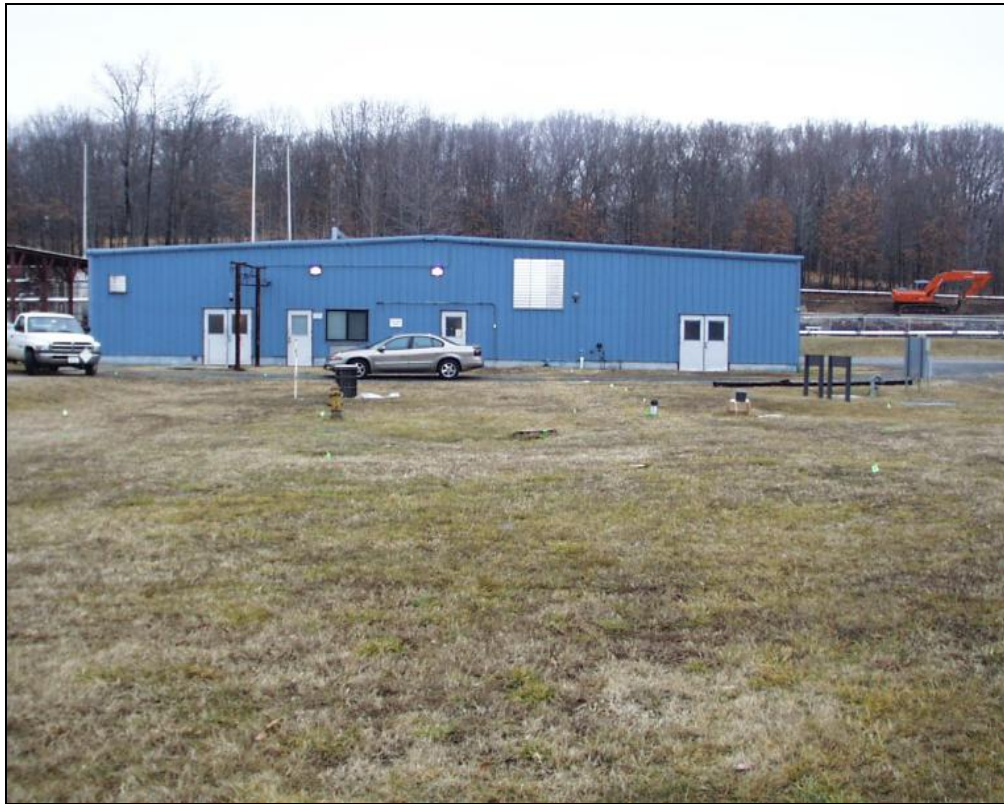
Figure 4-1. Location of the Raman Sensor Field Demonstration at the IHDIV Site.
