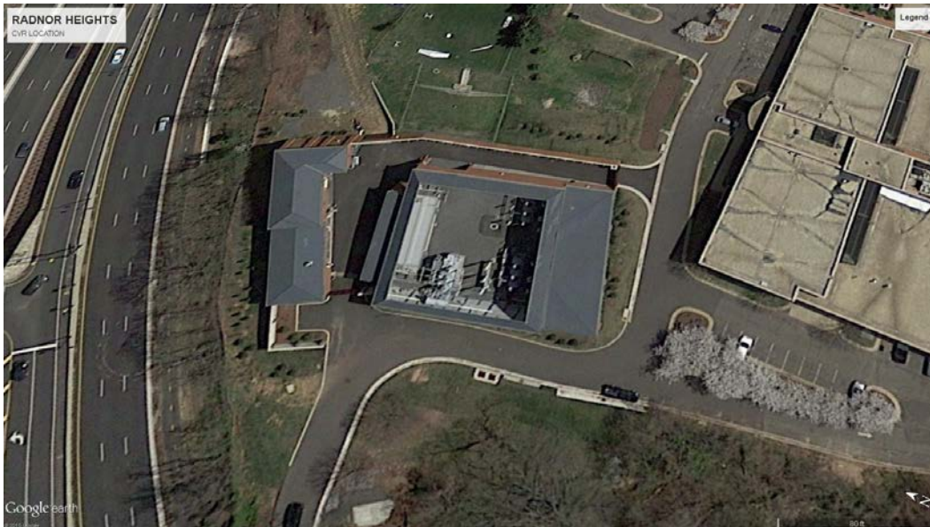
Figure 15. Aerial Picture of Radnor Heights Substation
