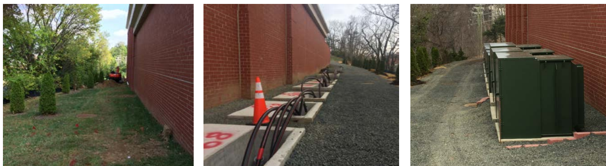
Figure 45. Single Phase Voltage Regulation Equipment Site Installations Conditions Prior, During, and at Completion on March 2016
