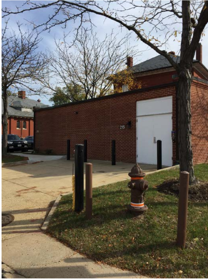
Figure 19. CVR and MicroCVR Observation Building 215
