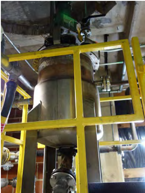
Lacquer Preparation Vessel
