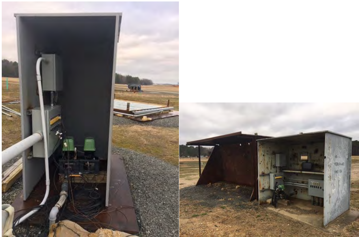
Figure 5. Shelter for the fuel delivery and pressure regulation system equipment and shelters for propane tank and fuel
