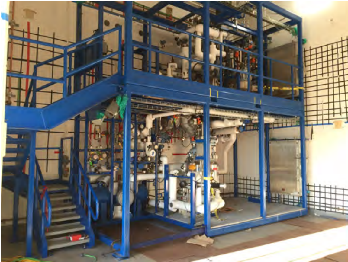
Figure 4 Pilot skid installed at LLNL Site 300.
