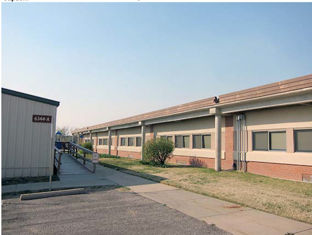
Photo (date): 6344J.JPG (taken 4/4/2016) Caption: South elevation, view to north
