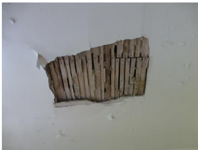
Exposed lath in the ceiling of Room 110. (Photo: CERL, 5/2/17)
