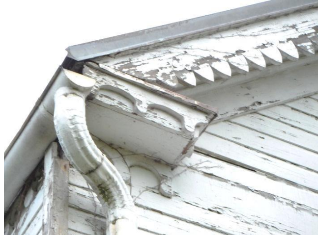
Fascia and cornice returns on the north elevation of the ell addition. (Photo: HPTC, 5/2/17)
