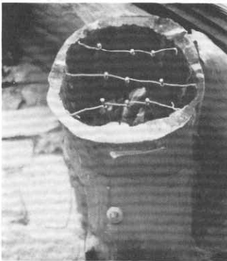
Illus. 17. Care must be taken to ensure that the replacement materials will work within a predesigned system. At the Norris Museum, Yellowstone National Park, the 12-inch diameter log rafters, part of an intricate truss system, had rotted at the inner core from the exposed ends back to a depth of 48 inches. The exterior wooden shells remained intact. Fiberglass rods (left photo) and specially formulated structural epoxy were used to fill the cleaned out cores and a cast epoxy wafer end with all the detail of the original wood graining was laminated onto the log end (right photo). This treatment preserved the original feature with a combination of repair and replacement using substitute materials as part of a well thought out system. Photos: Courtesy of Harrison Goodall.
