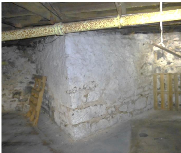
Whitewashed masonry main block foundation and triangular west elevation chimney foundation. (Photo: CERL, 5/2/17)
