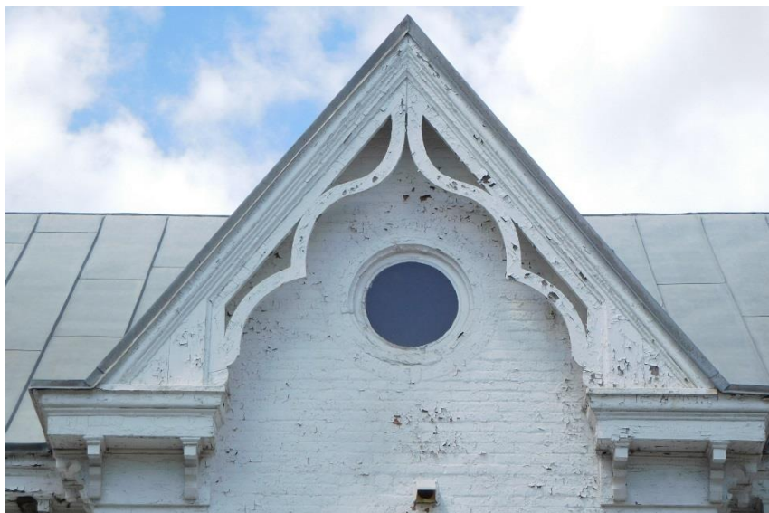
An oculus window with Plexiglas lite on the south elevation. (Photo: HPTC, 5/2/17)
