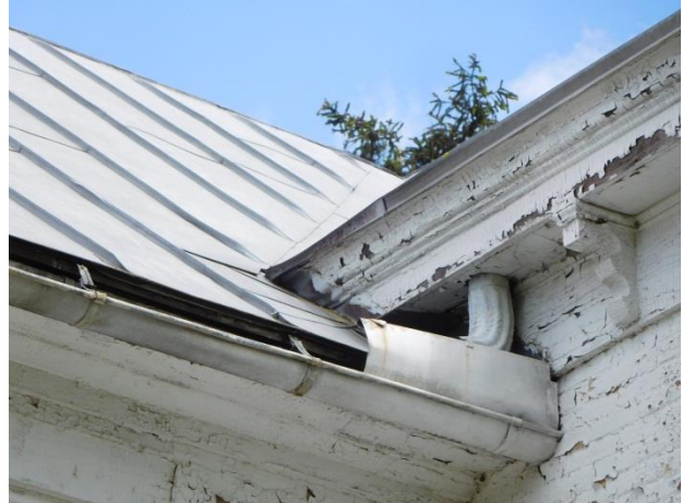
Half-round gutter on the ell addition and box gutter on the main block. (Photo: HPTC, 5/2/17)
