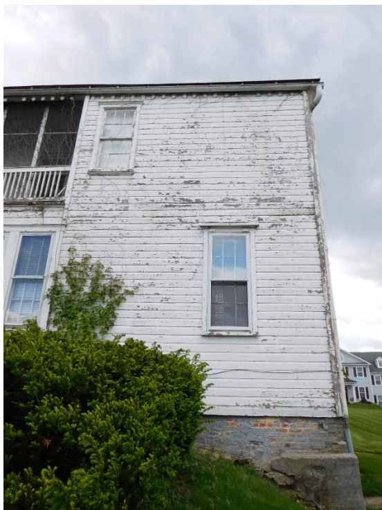
East elevation of the ell addition with painted wood novelty siding. (Photo: HPTC, 5/2/17)
