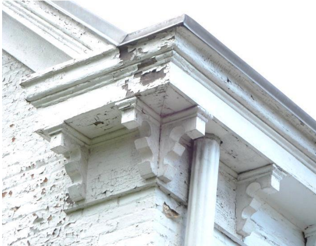
Wood cornice and brackets on the main block. (Photo: HPTC, 5/2/17)
