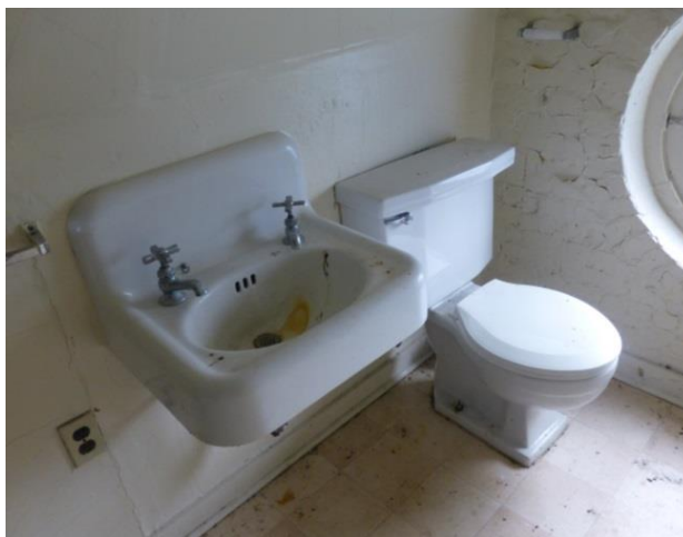
Sink and toilet in the third-floor bathroom (Room 301). The sink is the only extant historic plumbing fixture in the building, but does not date to the period of significance. Note also non-historic baseboards. (Photo: CERL, 5/2/17)
