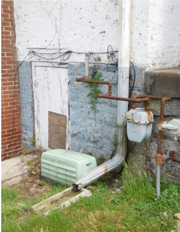
Downspout with splash pad, northwest corner of ell addition. (Photo: HPTC, 5/2/17)
