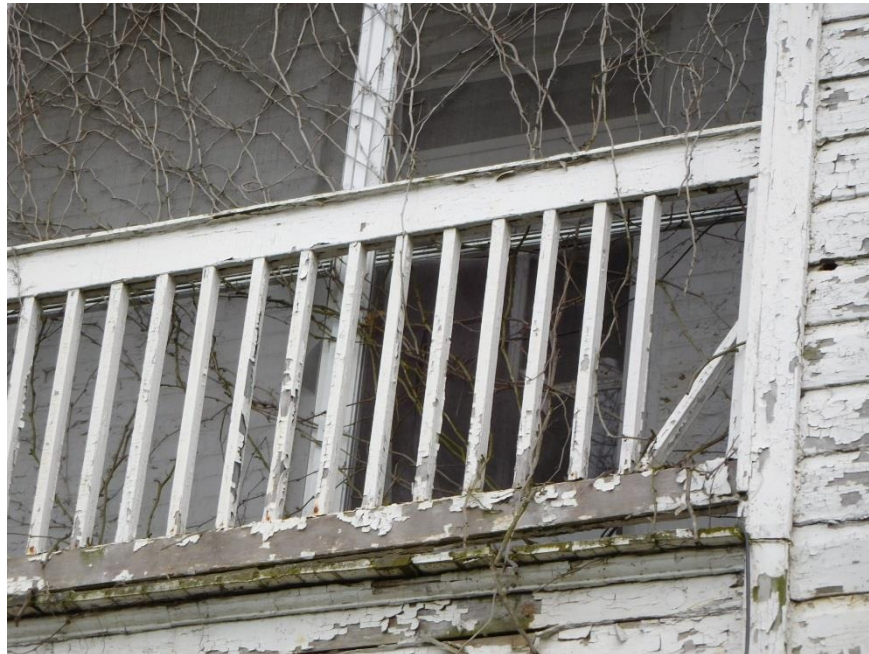
The second-floor balcony railing on the east elevation of the ell addition has damaged wood components and significant paint failure. (Photo: HPTC, 5/2/17)
