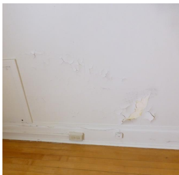
Most wall finishes in Unit B are historic plaster. Note paint failure. (Photo: CERL, 5/2/17)
