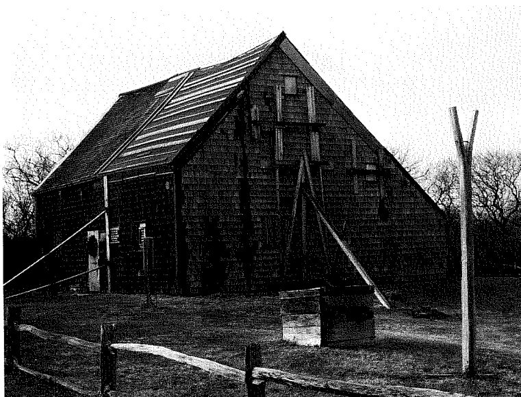
Figure 3. Buildings seriously damaged by storms or deterioration may need to be braced before architectural evaluations can be made. Jethro Coffin House. Photo: John Milner Architects.
