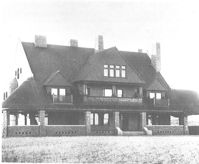
These two views of the same house demonstrate how the use of a substitute material can drastically affect the overall character of a structure. The textural interest of the original tile roof was lost with the use of asphalt shingles. Recent preservation efforts are replacing the tile roof. (Frank House, Kearney, Nebraska, photo courtesy of the Nebraska State Historical Society, Lincoln, Nebraska)
