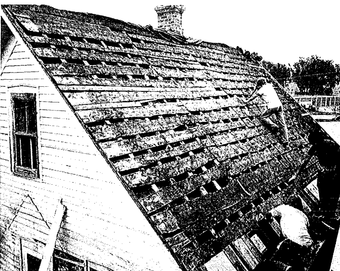
7. The reshingling of the circa 1856 Stovewood House in Decorah, Iowa, revealed the original open sheathing boards and pole rafters. Sawn cedar shingles were used as a replacement for the historic cedar shingles seen still in place at the ridge. A new starter course is being laid at the eaves. Photo: Norwegian-American Museum, Decorah, Iowa.
