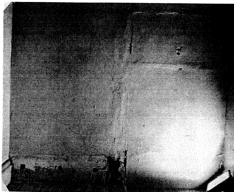
Figure 9. Raking light is used to show irregularities on flat surfaces. Patches, repairs, and alterations can then be mapped by the shadows or ghosts they cast. In this case, the pattern of patched plaster suggested the removal shelves and a balustrade handrail from the wall. Historical research and plaster analysis confirmed the findings and the sequence of change.
