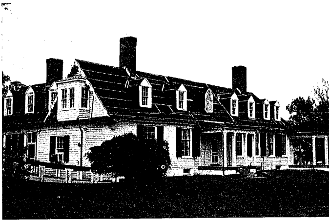
A. The later non-historic shingles were removed from Appomattox Manor (circa 1840 with later additions) and roofing paper was installed for temporary protection during the re-shingling.
