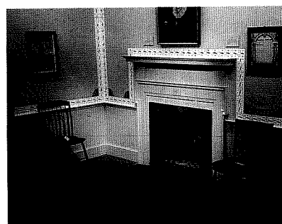
Figure 2. The paint chronology of this mantel, seen in the exposed paint layers in the left corner, proved it had been relocated from another room of the house. To remove a significant feature's paint history and the evidence of its original sequence of color by stripping off all the paint is inappropriate — and unnecessary — as part of a lead hazard reduction project. Careful surface preparation and repainting with lead-free top coats is recommended. Photo: NPS Files.
