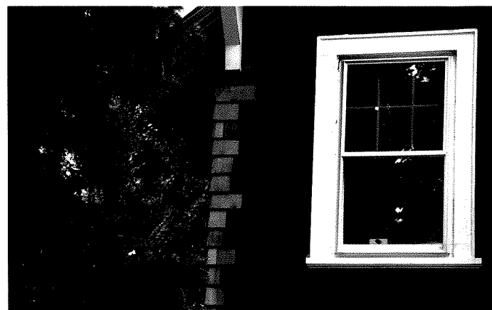
Figure 7. One of the advantages of wood shingles as a wall covering is that individual shingles that are damaged can easily be replaced. On this highly exposed corner, worn shingles have been selectively replaced to help safeguard against water damage. The new shingles will be stained to match the existing shingles.
