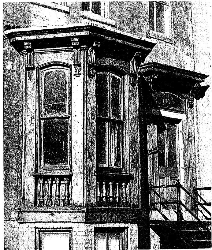
Fig. 2 A traditionally painted bay window has been stripped to bare wood, then varnished. In addition to being historically inaccurate, the varnish will break down faster as a result of the sun's ultraviolet rays than would primer and finish coats of paint. Photo: David W. Look, AIA.
