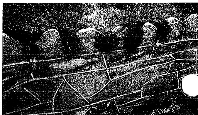
Figure 20. This stone garden wall was tuckpointed to match the tuckpointing on the c. 1920s house on the property. Photo: Anne Grimmer.
