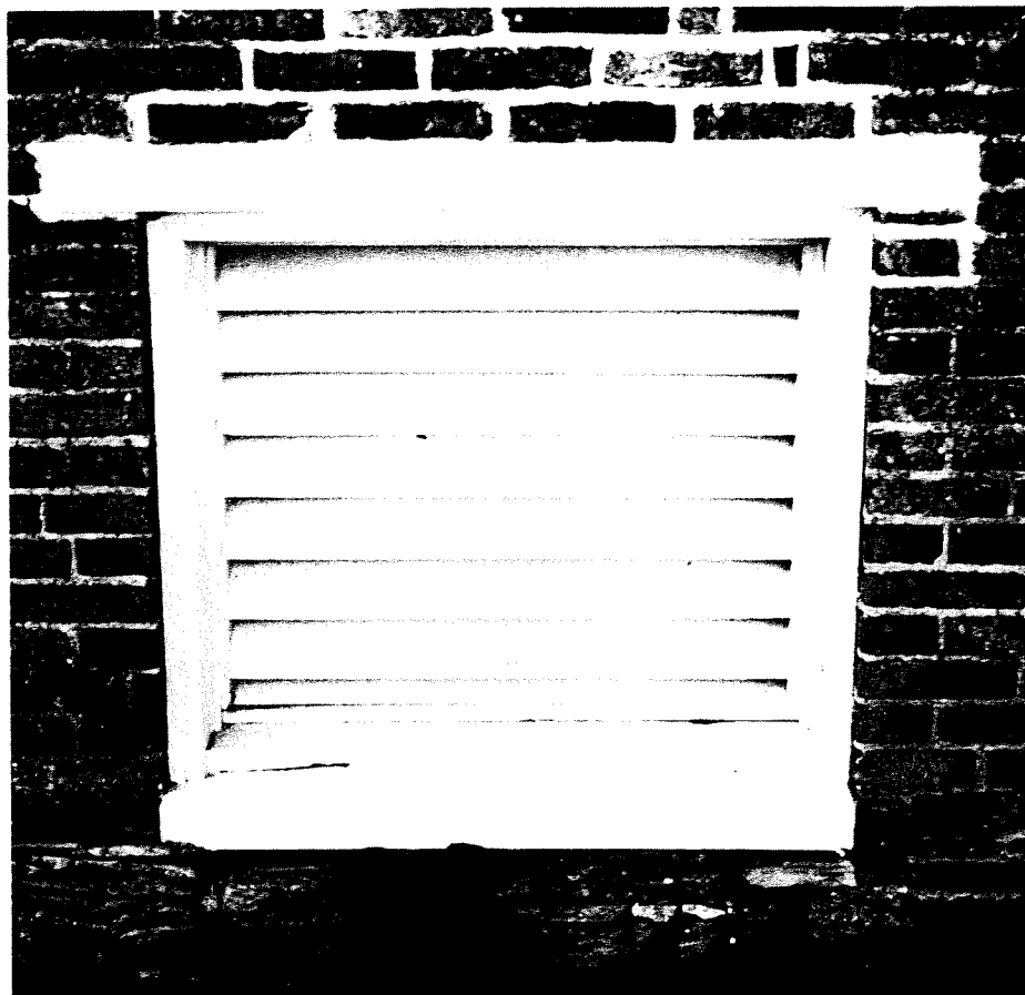
Figure 1. Full louvered vents were installed in all single-sash openings in the basement because of the more severe moisture problems present in that location. Photo: Charles Fisher
