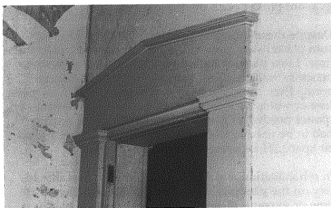
Fig. 5 (a). The photo above shows the use of wooden plaster “grounds” nailed to the wall studs of the mid-19th century Lockwood House in Harpers Ferry, West Virginia. This allowed the plasterer to work flush with the surface of the grounds. Afterwards, the carpenter could nail the finish woodwork to the ground, effectively hiding the joint between the plaster and the ground. The trim was painted after its installation, leaving a paint outline on the plaster. Fig. 5 (b). The photo below shows door trim and mouldings in place after the plastering was complete. Photos: Kaye Ellen Simonson.
