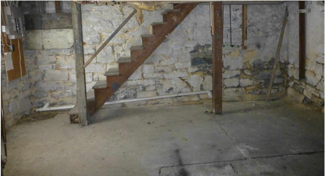
Unfinished concrete slab on grade in the basement of Unit B (Room 003). (Photo: CERL, 5/2/17)
