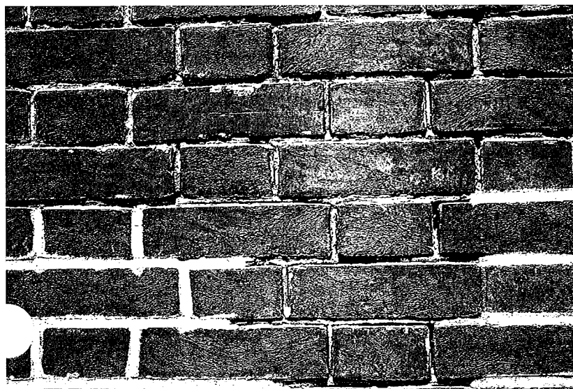
Figure 4. (left) The poor quality of this repointing—it appears to have been “tooled” with the mason’s finger—does not match the delicacy of the original beaded joint on this 19th-century brick wall. (right) It is obvious that the repointing on this “test patch” is not an appropriate replacement mortar joint for this early-19th century stone foundation. Photos: Lee H. Nelson, FAIA.
