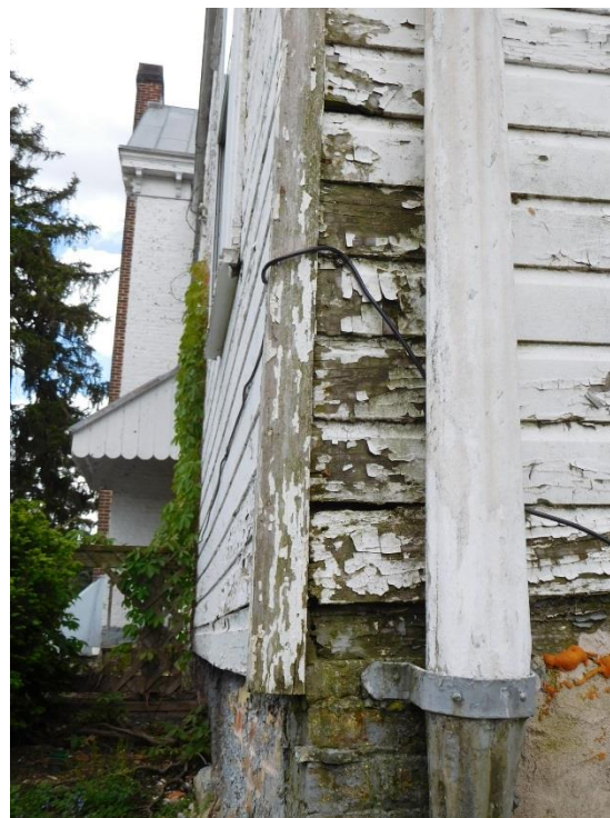
Paint failure and deterioration at the northeast corner of ell addition. (Photo: HPTC, 5/2/17)
