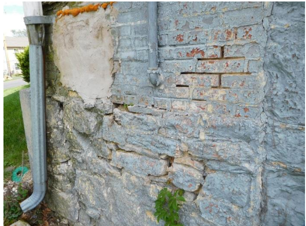
The southwest corner of the ell foundation has concrete and brick patches and missing mortar joints. (Photo: HPTC, 5/2/17)
