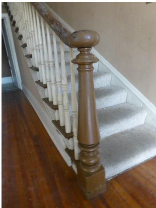
Historic newel post and balustrade on the main stairs in Unit A. (Photo: CERL, 5/2/17)
