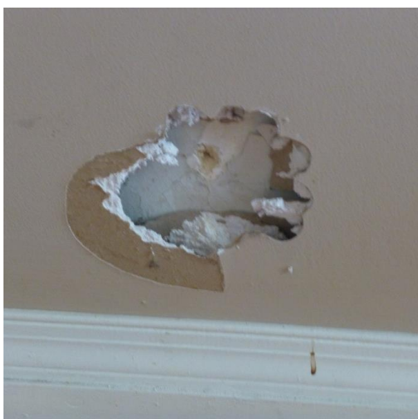
Damaged drywall walls in Room 304 in Unit A. (Photo: CERL, 5/2/17)
