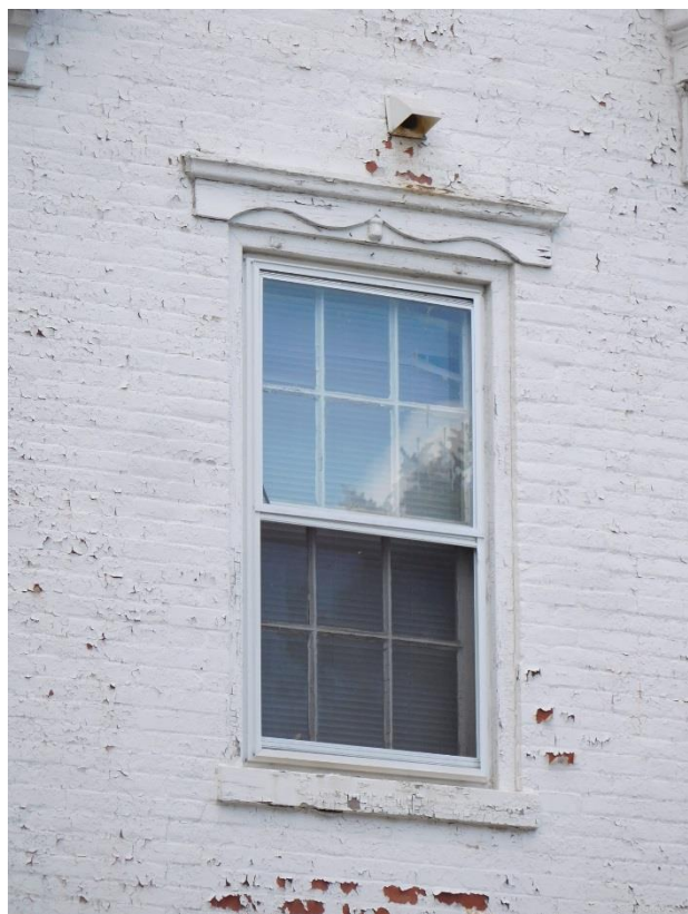
Typical historic wood 6-over-6 double-hung window on the south elevation with a decorative hood and an exterior storm unit. (Photo: HPTC, 5/2/17)
