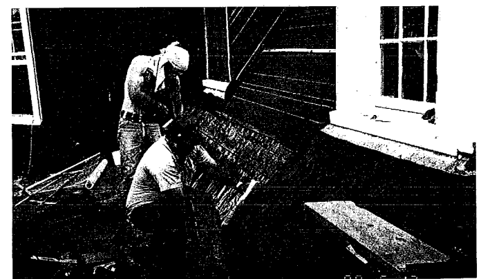
E. In order to achieve a "Class B" fire-rating, the shingles were dipped in fire-retardant chemicals and allowed to dry prior to installation. Iron oxide was added to this chemical dip to stain the shingles to match the historic red color. These coatings will need periodic reapplication.
