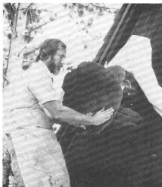
Illus. 17. Care must be taken to ensure that the replacement materials will work within a predesigned system. At the Norris Museum, Yellowstone National Park, the 12-inch diameter log rafters, part of an intricate truss system, had rotted at the inner core from the exposed ends back to a depth of 48 inches. The exterior wooden shells remained intact. Fiberglass rods (left photo) and specially formulated structural epoxy were used to fill the cleaned out cores and a cast epoxy wafer end with all the detail of the original wood graining was laminated onto the log end (right photo). This treatment preserved the original feature with a combination of repair and replacement using substitute materials as part of a well thought out system. Photos: Courtesy of Harrison Goodall.
