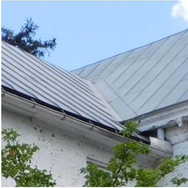
Valley flashing between the ell addition and main block roofs. (Photo: HPTC, 5/2/17)
