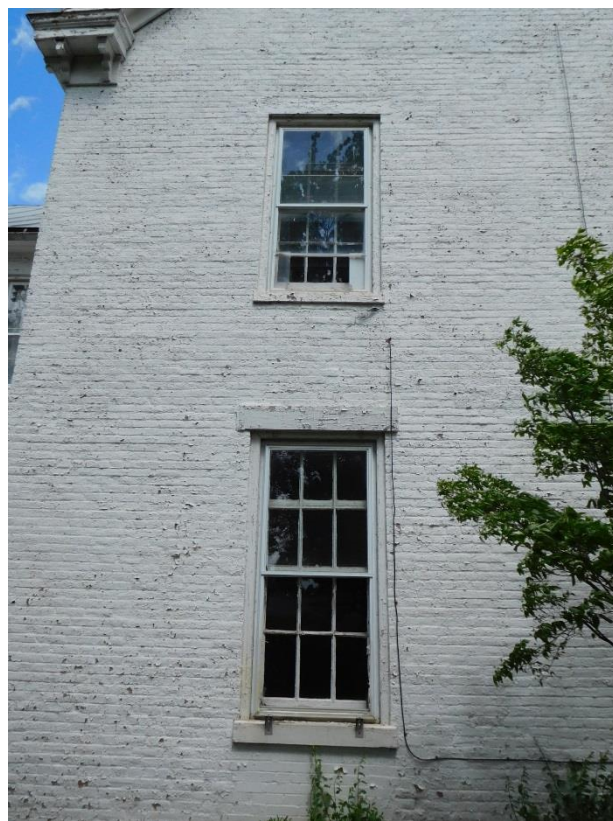
Typical windows on the west elevation of the main block with plain wood lintels and sills. (Photo: HPTC, 5/2/17)
