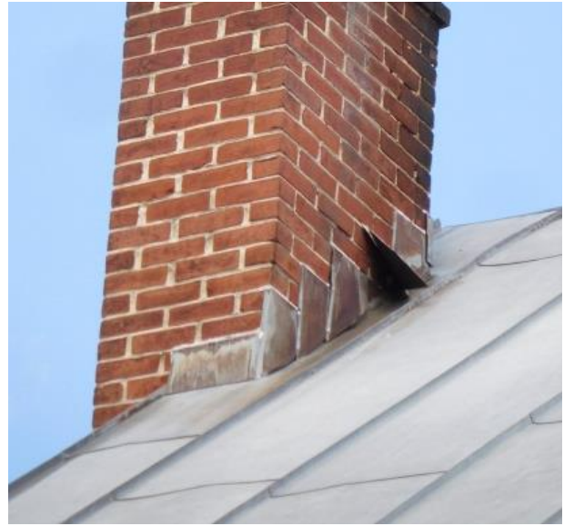
The step flashing has separated from the south chimney on the ell addition. (Photo: HPTC, 5/2/17)
