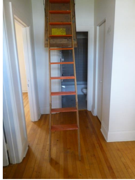
Attic access stair in Unit B (Room 204). The bottom tread is missing. (Photo: CERL, 5/2/17)
