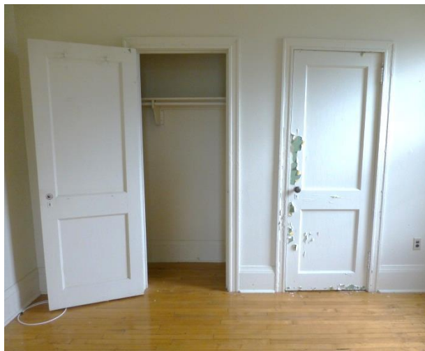
Closet doors, Room 202, Unit A. Most of the closet doors in Unit A are through-tenoned. Note that one door retains its historic hardware and one does not. (Photo: CERL, 5/2/17)
