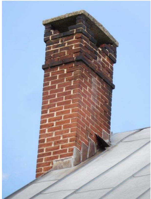
The step flashing on the north chimney on the ell addition has become loose. (Photo: HPTC, 5/2/17)
