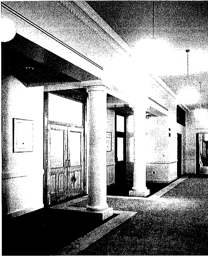
b. Central air conditioning was installed in the corridors of this circa 1900 school building by adding an air handler over the entrance from a vestibule. Custom-designed slot registers provide linear diffusers without detracting from the architecture of the space. Photo: Lautman Photography courtesy of Notter Finegold + Alexander Inc.
