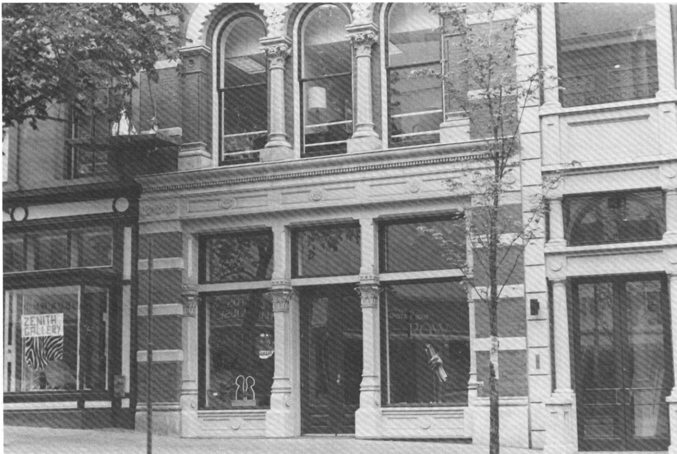
The new cast aluminum storefront replaced the lost 19th-century cast-iron original. Photo: Sharon C. Park, AIA.
