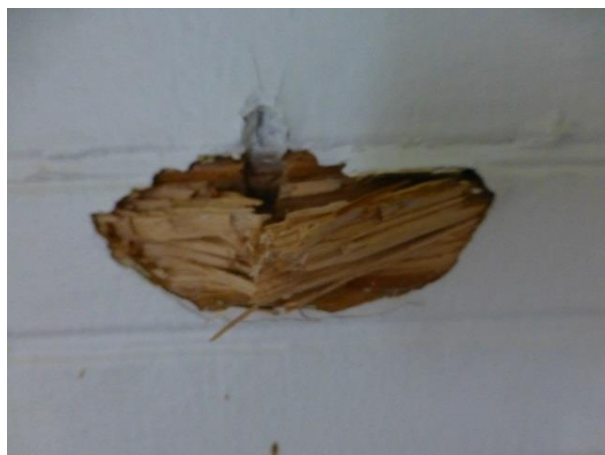
Beaded board wall finish damaged by invasive materials testing in Room 106. (Photo: CERL, 5/2/17)
