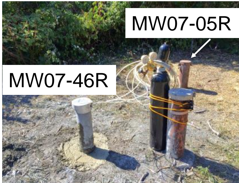
Figure 5.2. Newly Installed Well MW07-46R Shown in Proximity to Existing Well MW07-05R.
