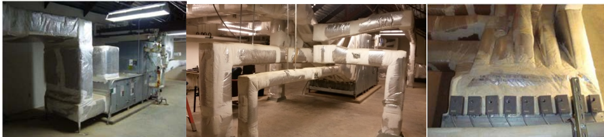
Figure 6. Example Air Handling Unit, Zone Ducts and Zone Actuators (at Fort Bragg)
