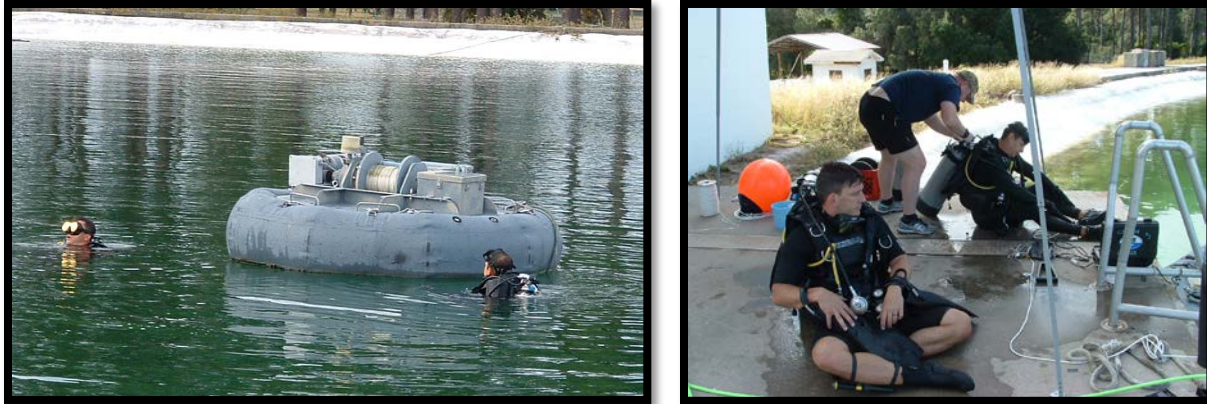
Figure 6. Inner-tube shallow water lift system and dive team for maneuvering system from within the water.
