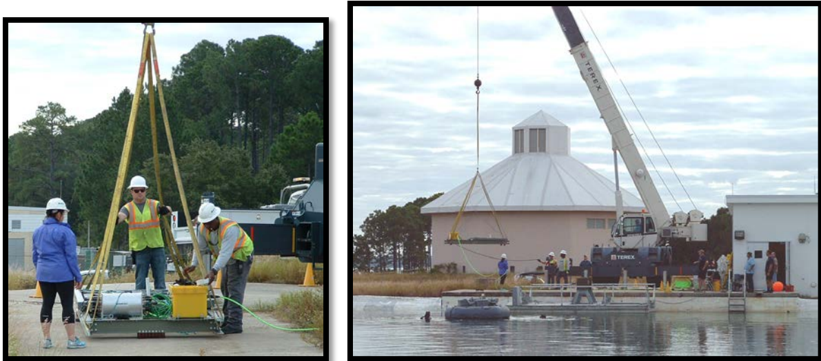
Figure 5. Crane provided by NSWPCD for transfer of system from land into water.
