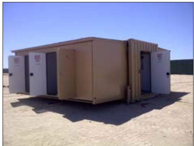
SuperCLU folding structure with easy set up and tear down; transported as an International Standards Organization container
