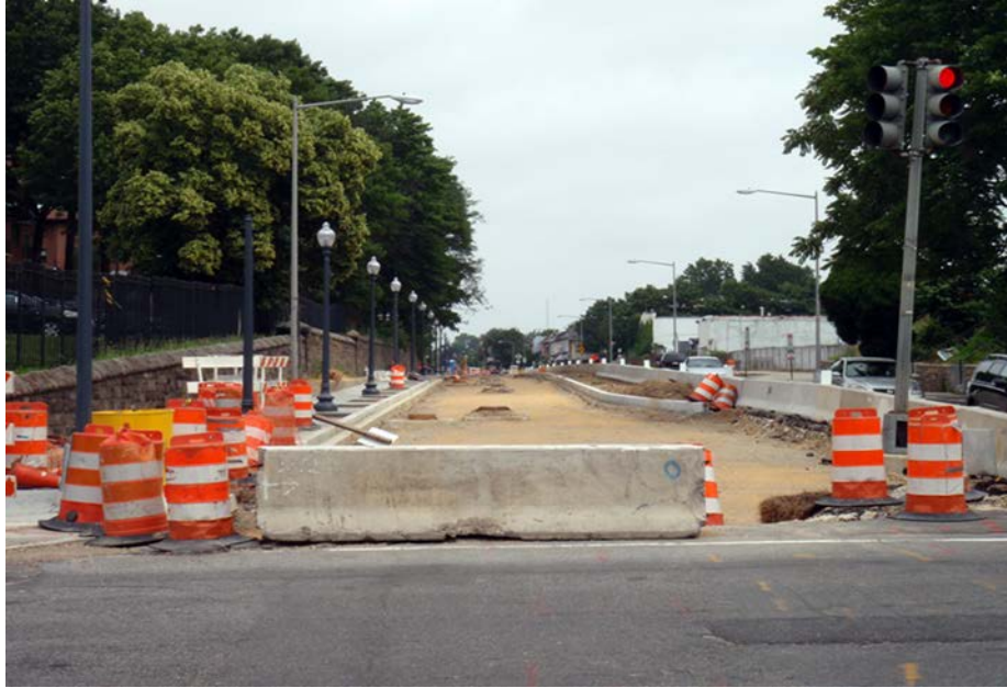
Figure 2. Temporary Concrete Barriers and Orange Plastic Traffic Barrels Used to Redirect Traffic for a Transportation Project in Washington, DC 40
