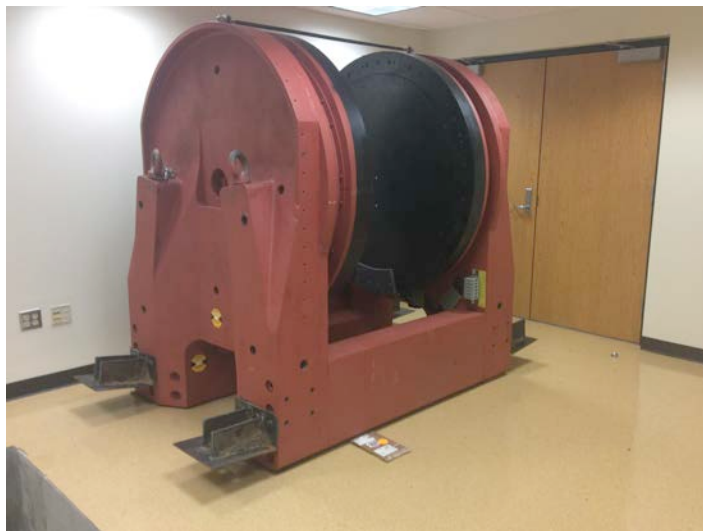
Figure 1. Clinical 15-ton 80-cm gap 0.05 T magnet during installation in Vanderbilt University Hospital building.
