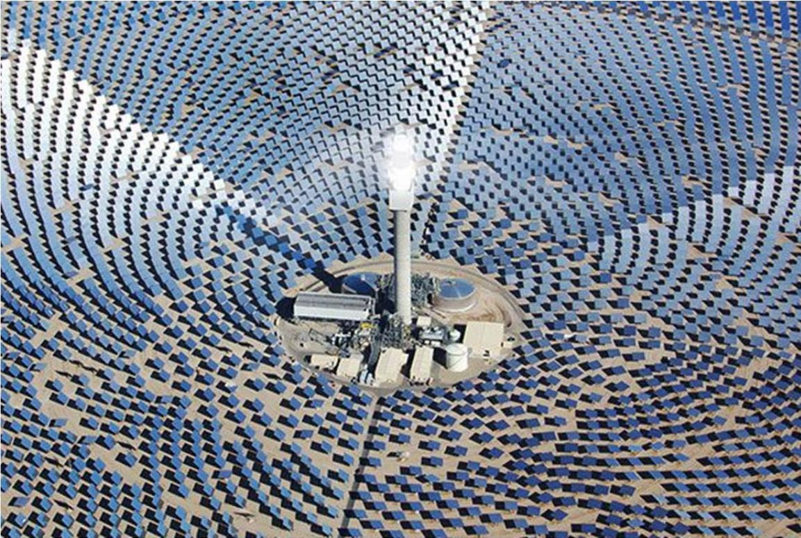
Figure 3. Centralized Solar Thermal Plant with Thermal Energy Storage.
