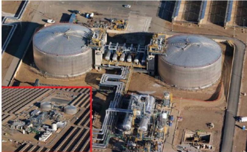
Figure 4. Andasol Parabolic Trough Solar Power Plant with Molten Salt TES. Source: [13].
