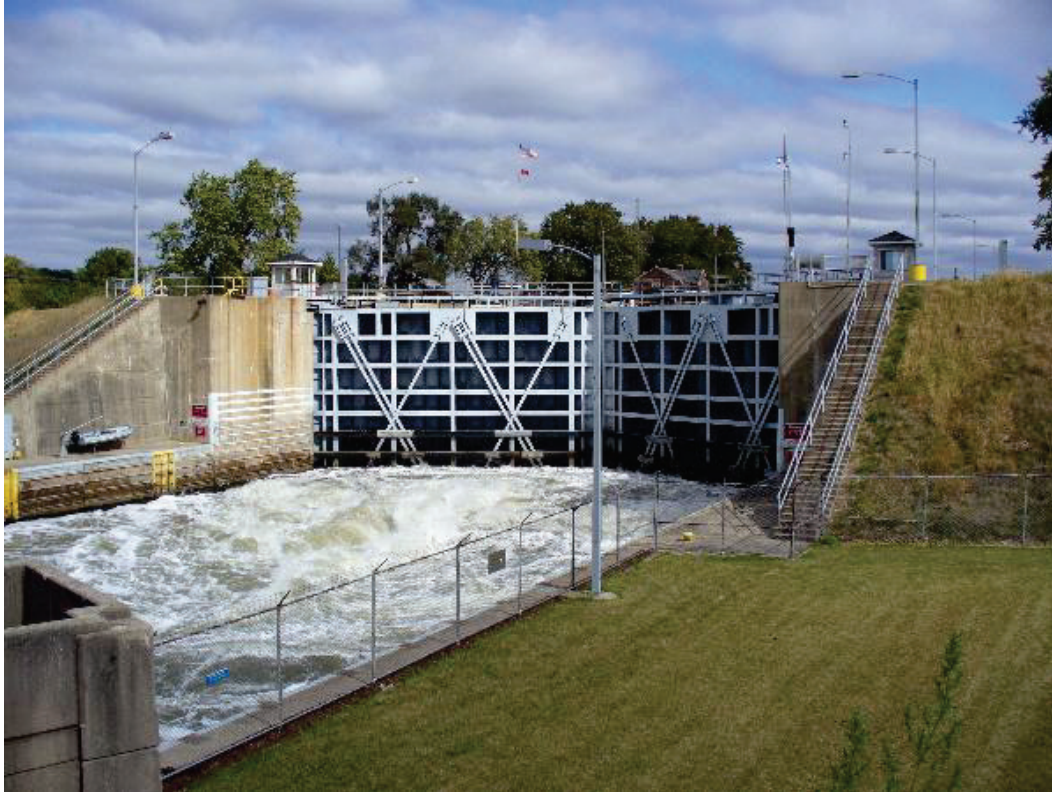
Figure 4. Picture taken during emptying of the navigation chamber at BRLD. Note highly turbulent conditions immediately downstream of the lock and for some distance downstream into the approach channel.
