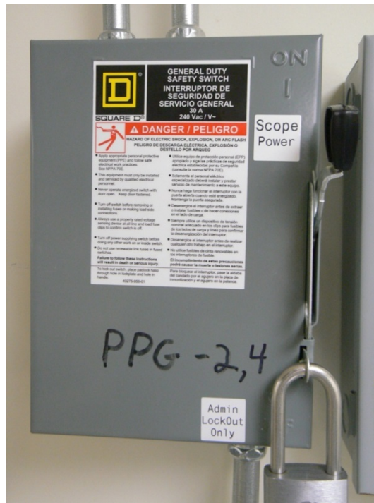
Figure 6-1: Main power for lift outlets, including telescope
