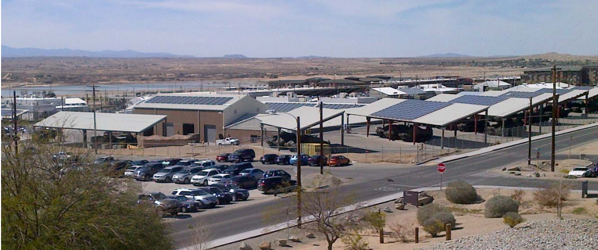
Figure 2. Photo of Equipment Garages with Rooftop Solar Installations at MCAGCC at Twentynine Palms, CA Showing Pole Mounted 12.5kV AC Distribution Network.
