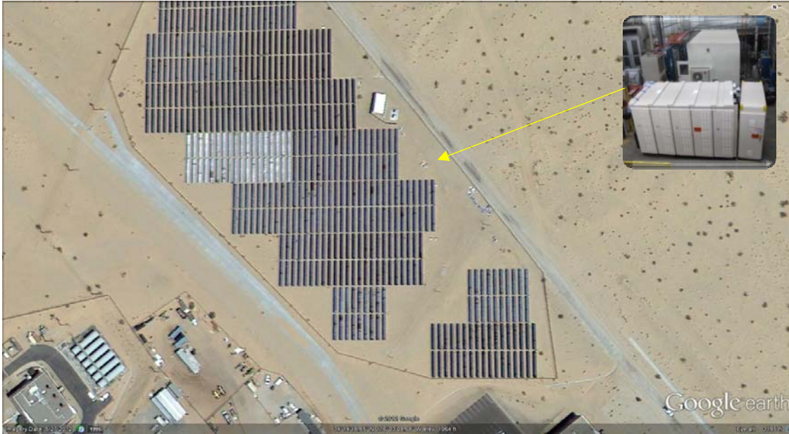
Figure 4. Aerial View of MCAGCC Solar Field with BESS Location Indicated.
