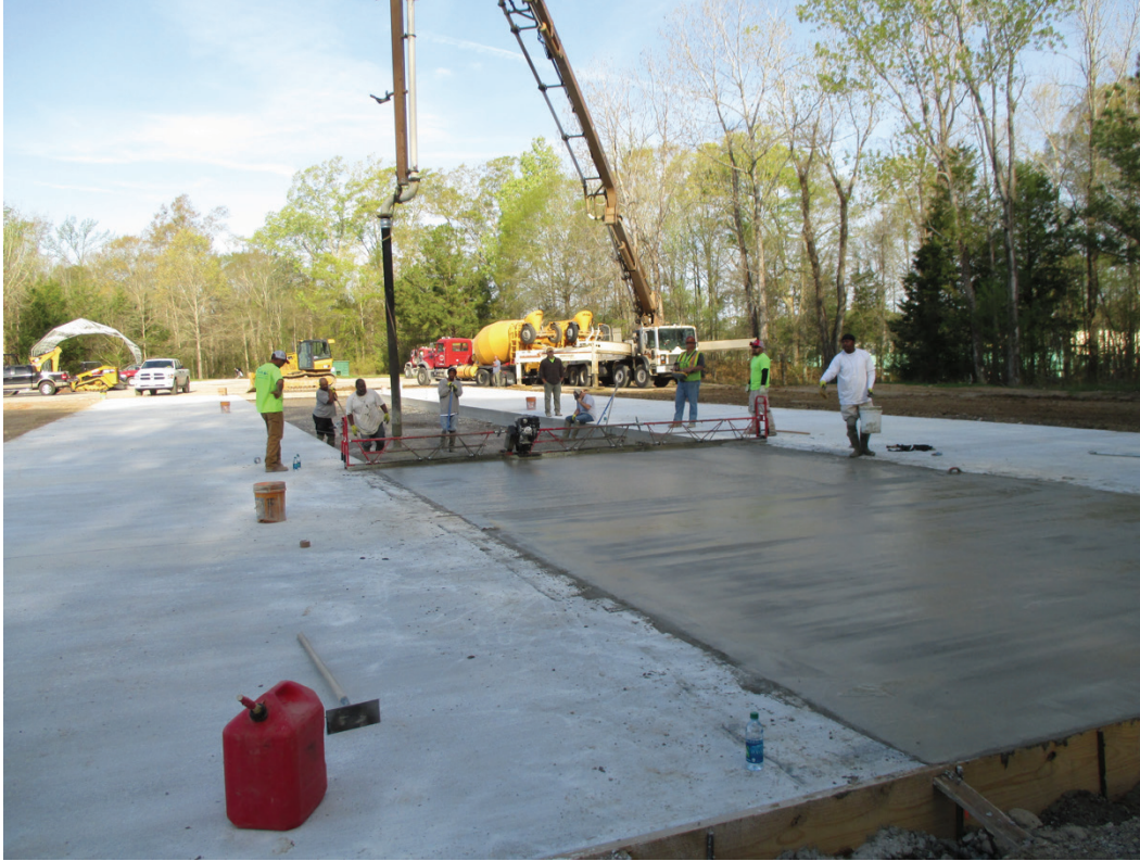
Figure 10. Placing and screeding PCC in Lane 2 using a pump truck.
