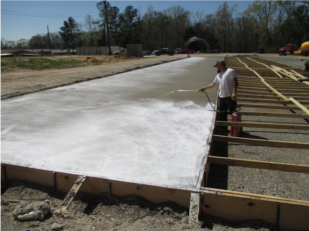
Figure 9. Applying curing compound to the PCC surface of Lane 3.
