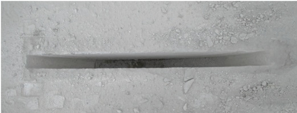
Figure 20. One plunge cut with the Caterpillar wheel saw attachment.
