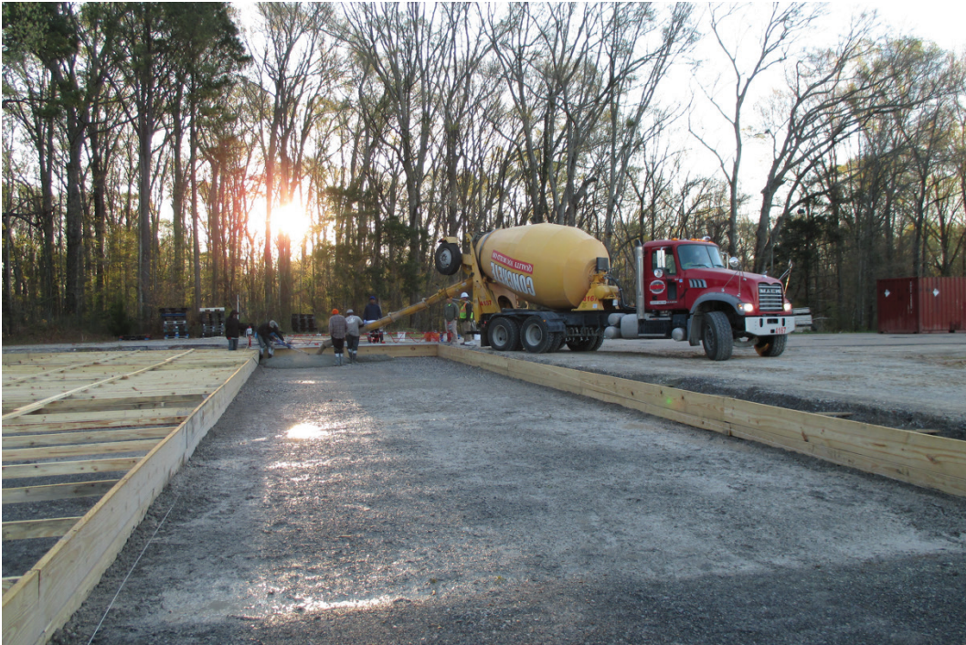
Figure 6. Placing PCC in Lane 3.
