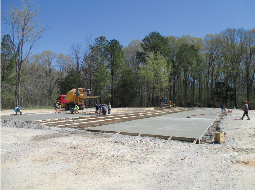
Figure 8. Finishing Lane 3 and placing and screeding PCC in Lane 1.
