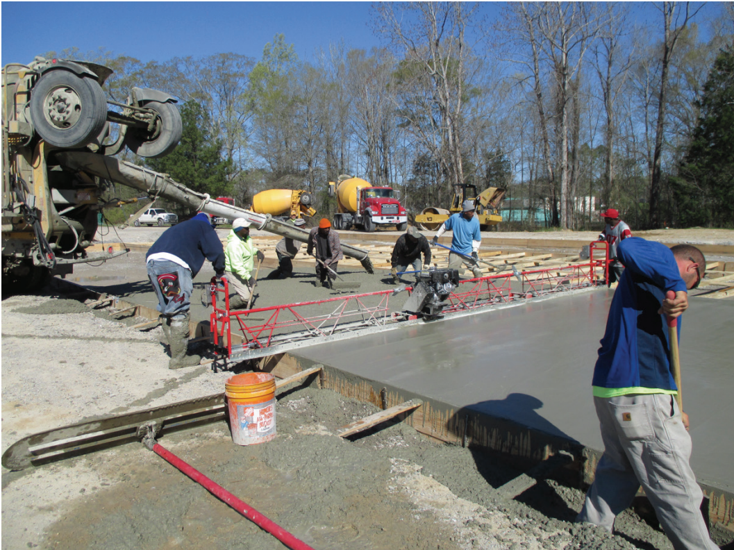
Figure 7. Using a vibratory truss screed and placing PCC in Lane 3.
