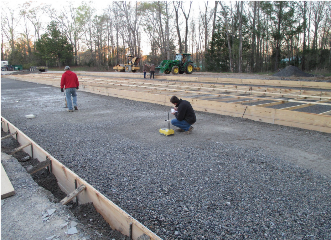
Figure 4. Measuring the density and moisture of the base layer using the nuclear density gauge.
