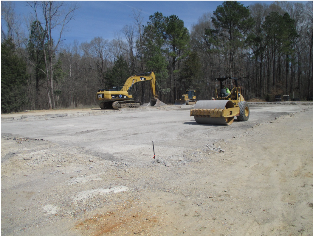
Figure 2. Compacting crushed limestone base material.
