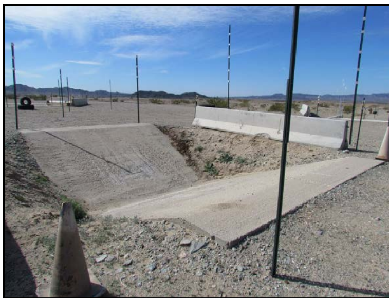
Figure 148. Direct approach V-ditch.
