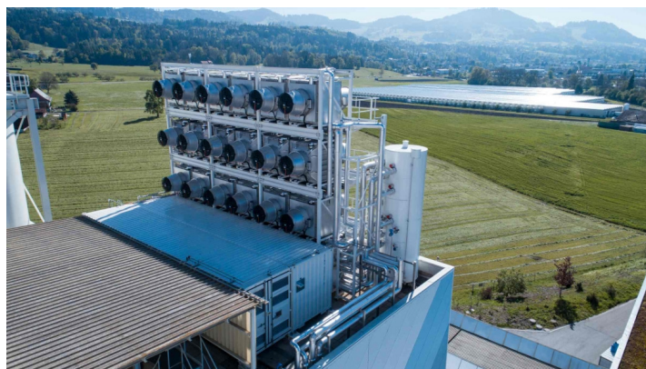
Swiss company Climeworks has developed the first commercial carbon capture plant. The facility scrubs carbon dioxide from the air and converts it to fertilizer. Source: www.climeworks.com
