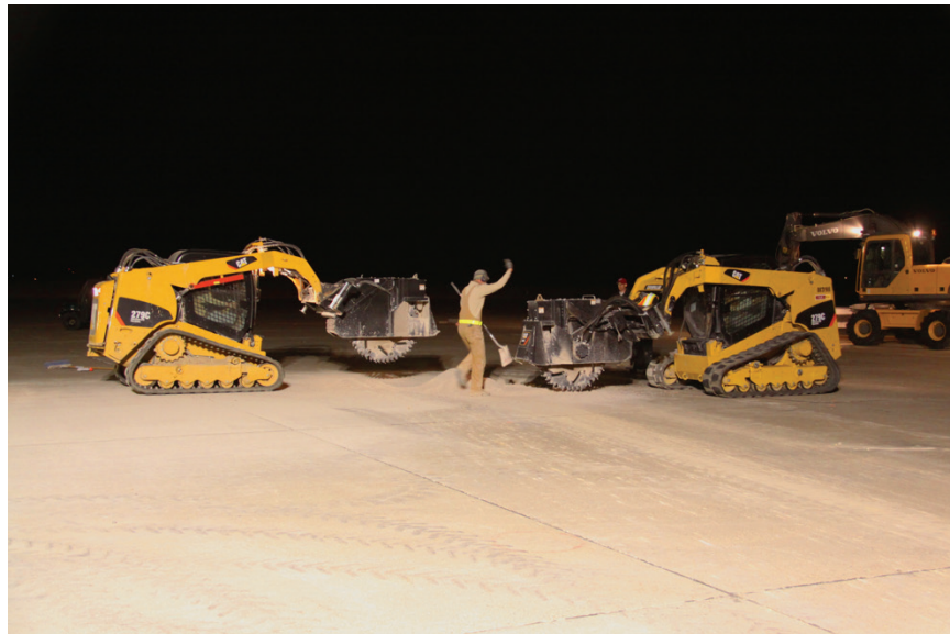
Figure 4. Saw cutting around crater upheaval.
