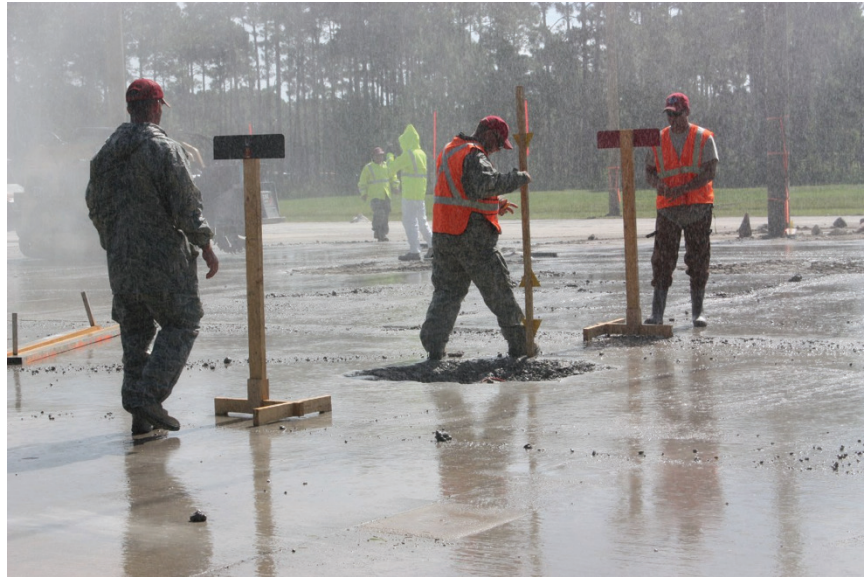
Figure 3. Crater profile measuring using stanchions.
