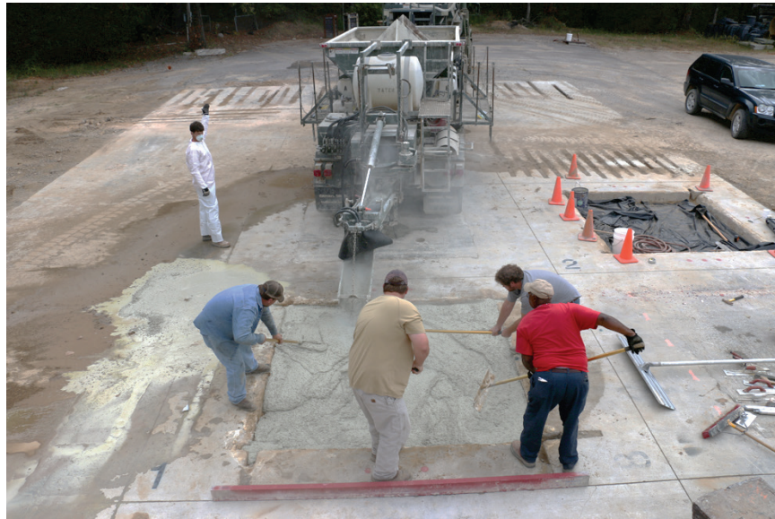
Figure 7. Crater repair with Rapid Set Concrete Mix® using the volumetric mixer.
