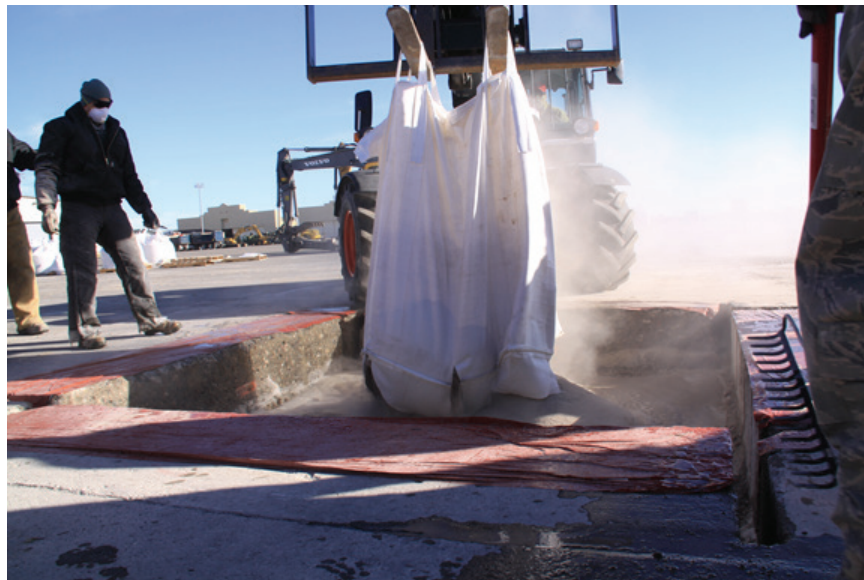
Figure 5. Placing flowable fill backfill using the dry method.
