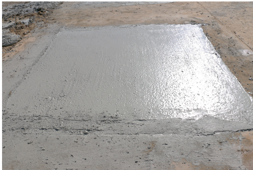
Figure 1. Rapid-setting concrete crater repair.
