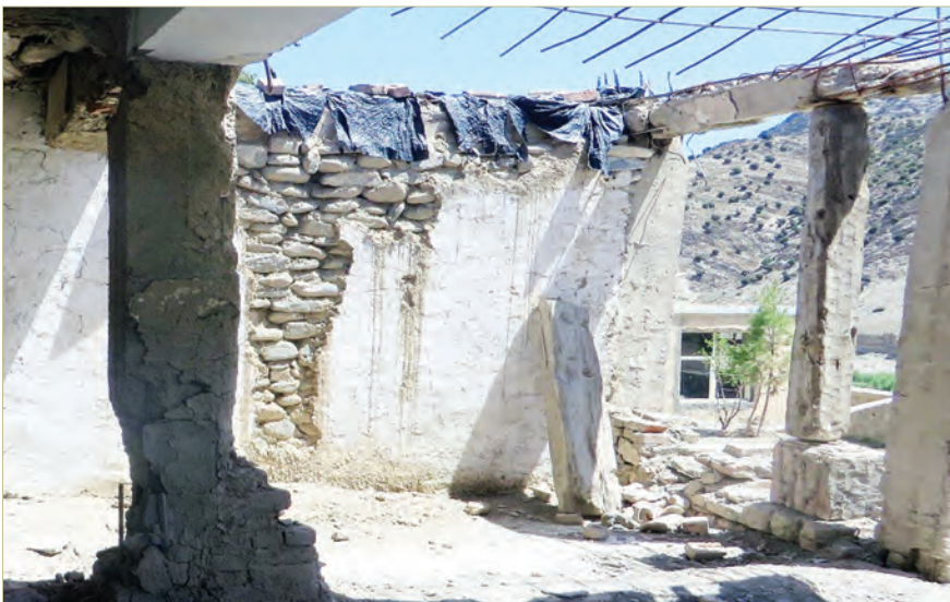
Construction at a Khowst Province health facility supported by USAID funds administered through a World Bank program. (SIGAR photo)
