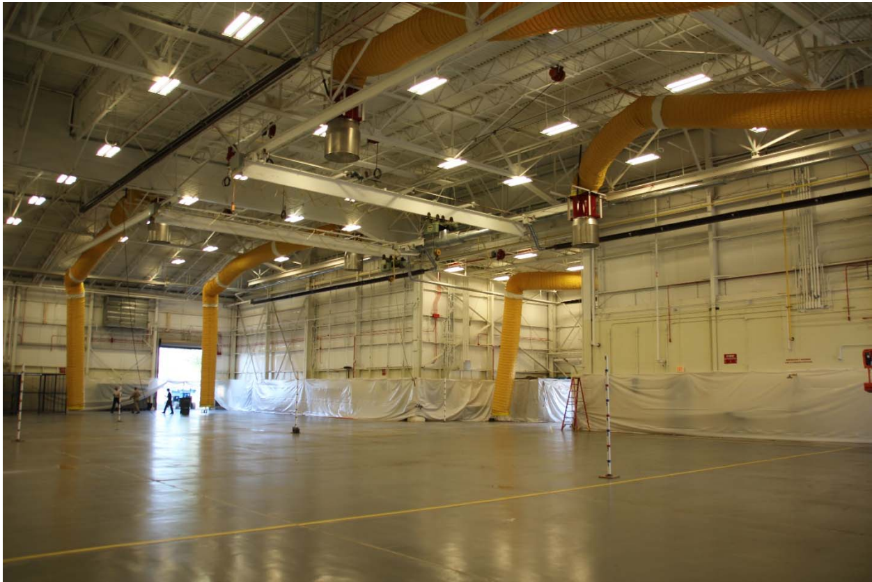
Figure 3. Protective Curtain on Hangar Boundaries
