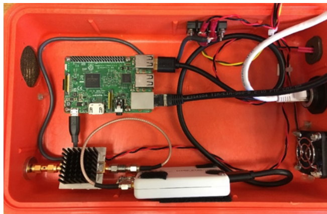
Fig. 9 SBC, SDR, and power amplifier installed in the bottom half
